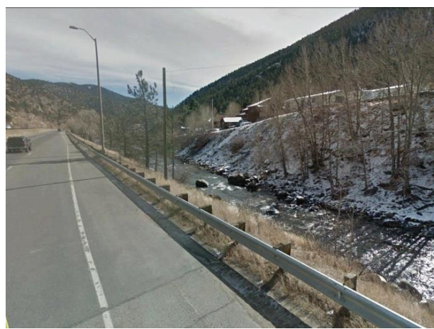
Eastbound I-70 runoff may drain directly to Clear Creek.
