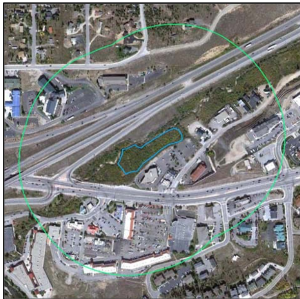
Figure 31 Aerial photograph of the Straight Creek AA (blue polygon) set in the context of the Surrounding Area (green polygon). Land use change has been substantial including retail and hospitality developments, infrastructure and low-density urban, but natural areas do remain. In this case the Surrounding Land Use Sub-variable was rate 0.61.
