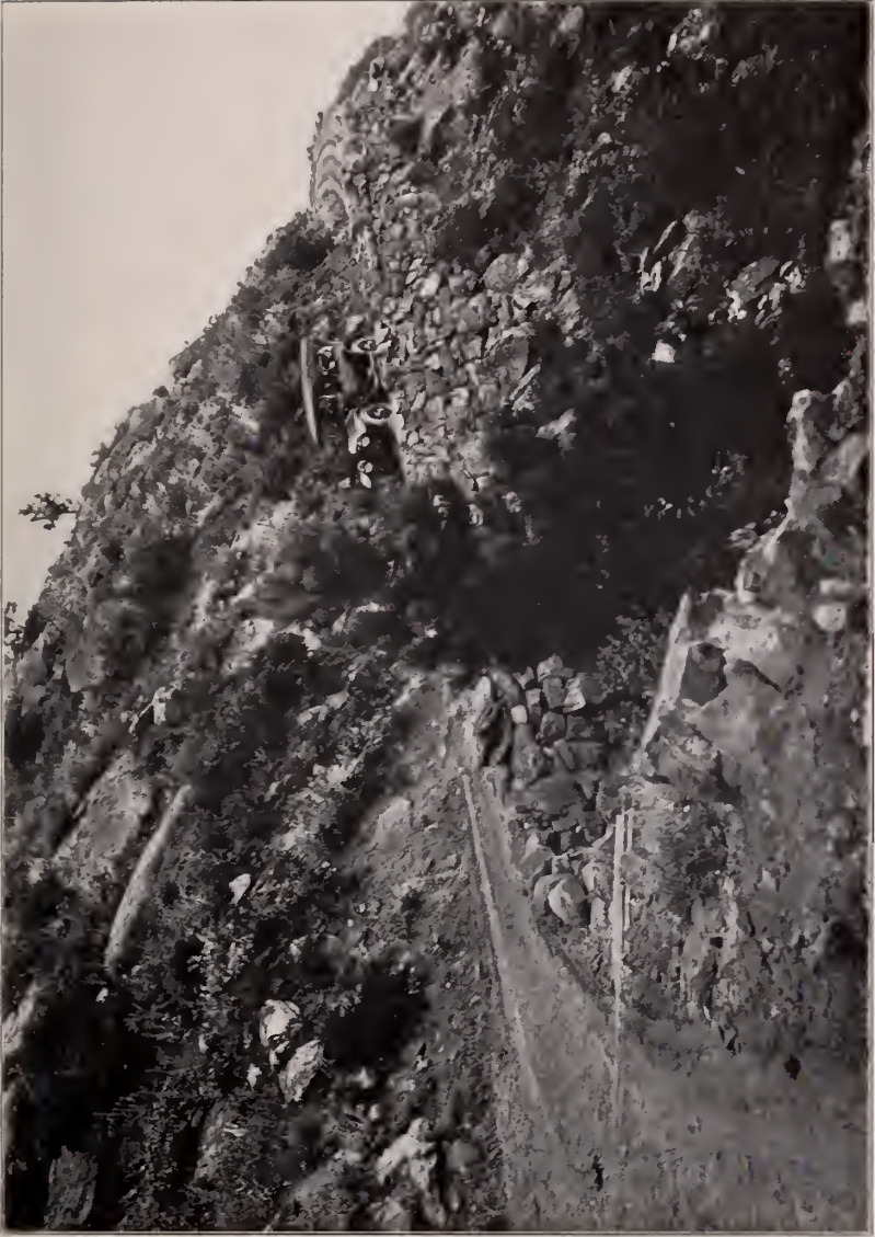
Completed Section of the Flagstaff Road, Near Boulder, Colorado
