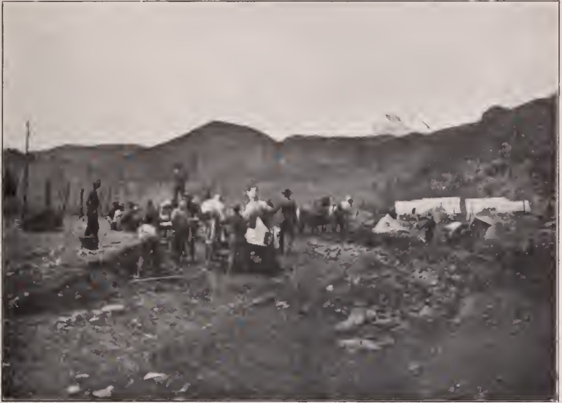
Another Section of the Stonewall Road. Work Prosecuted Under Supervision of Committee
