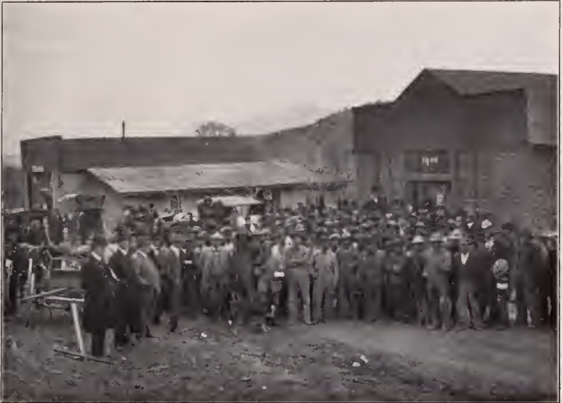
"Paying Off" 225 Men for Work on the Stonewall Road
