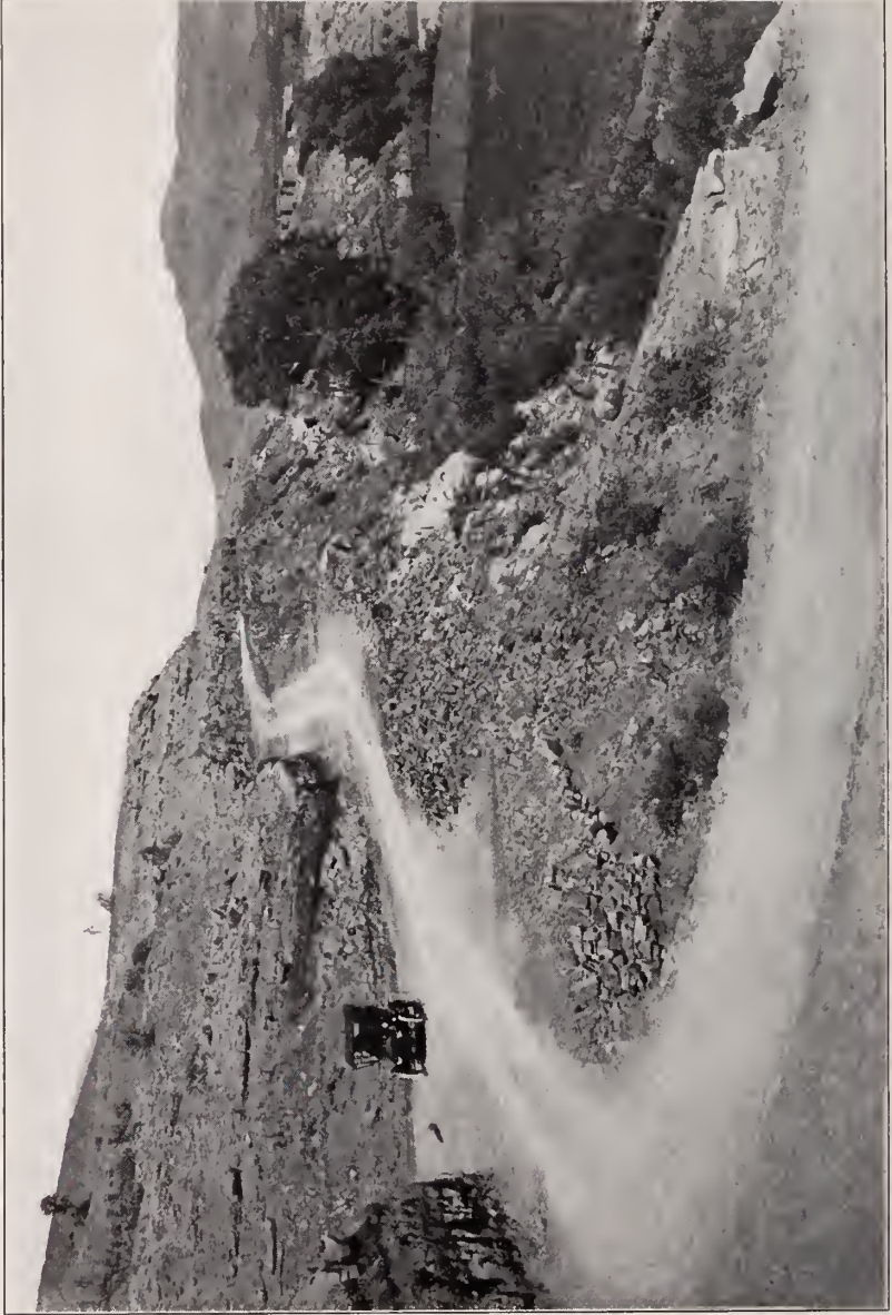
A Finished Section of the Stonewall Road. Work Prosecuted Under Supervision of Committee
