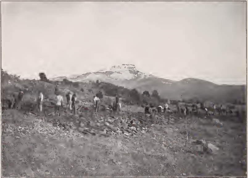
Santa Fe Trail, Near Trinidad, Colorado. Fisher's Peak in Background. Work Prosecuted Under Supervision of Committee
