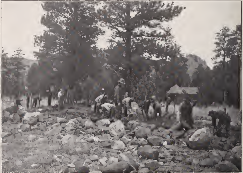
Pioneer Work on Stonewall Road, Near Trinidad. Mr. Radford's Cottage in Right Background. Work Prosecuted Under Supervision of Committee
