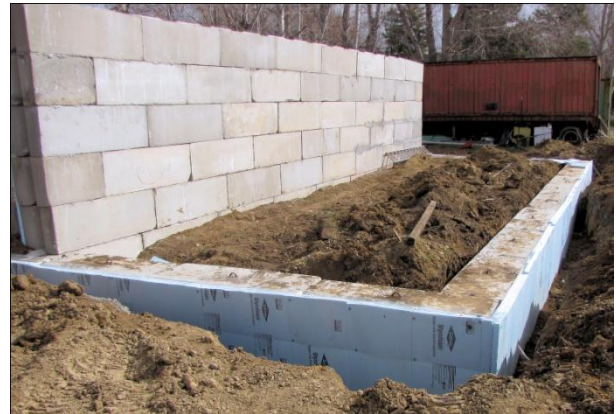
Figure 2-3. Foundation and north wall of research greenhouse.
