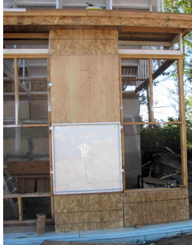
Figure 3-14. Pocket shutter installed.
