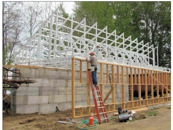
Figures 3-7 and 3-8. These trusses were lifted in place by a 1947 vintage hay loader.
