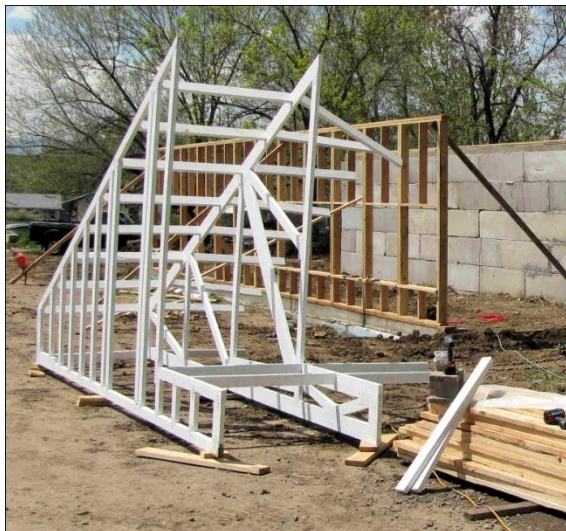
Figures 3-7 and 3-8. These trusses were lifted in place by a 1947 vintage hay loader.
