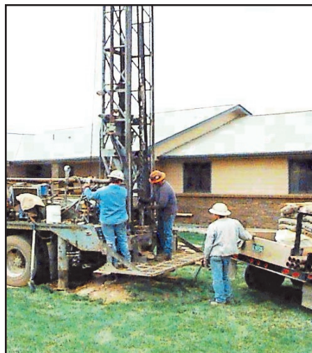
Well construction near Northglenn
