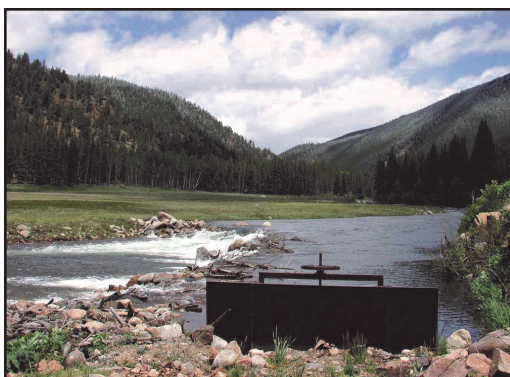
Diversion Structure on Crystal Creek
