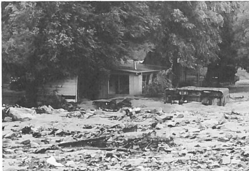
DAMAGE FROM SEDIMENTATION BIG THOMPSON CANYON
