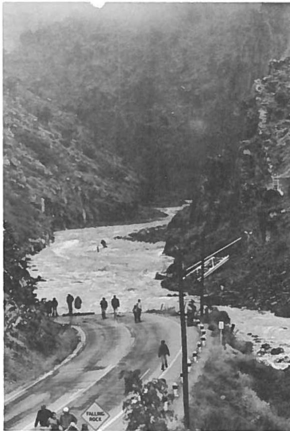
DESTRUCTION OF HIGHWAY 34 BIG THOMPSON CANYON
