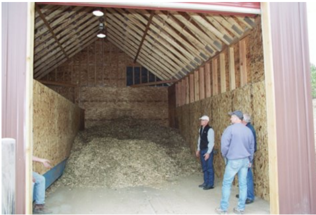
Figure 2.2 Fuel Storage Building
