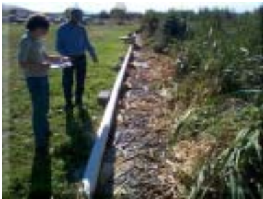
Inlet pipe to wetland cells
