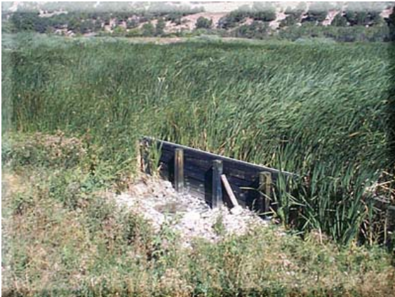
Levees with removable boards
