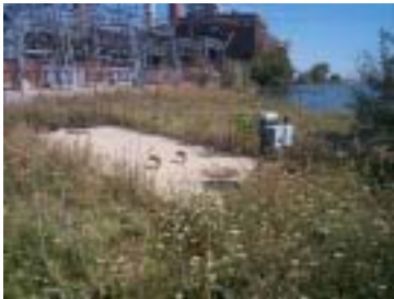
Septic tank that precedes the wetland cells
