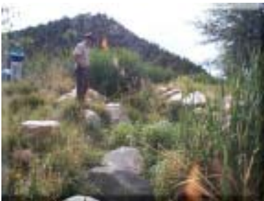
A cobbled pathway serves as an overflow structure to connect the wetland cells
