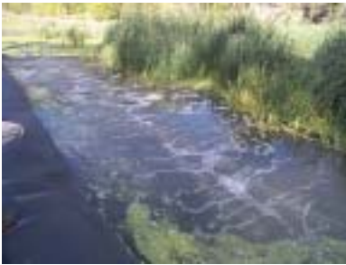
Aerated influent end of wetland
