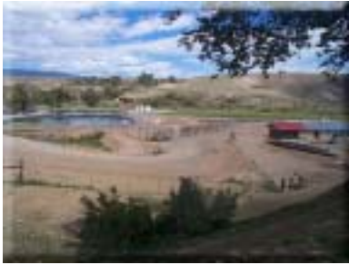
Overview of Wastewater Treatment Facility
