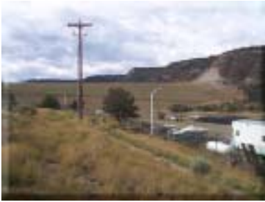
Overview of the Wastewater Treatment Facility
