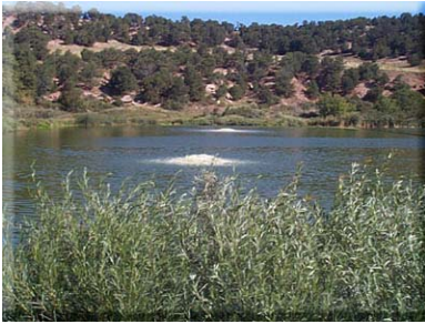
View of aerated lagoon
