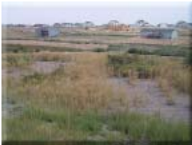
Subsurface Flow Wetland Cell
