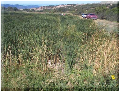
Perimeter of wetland cell
