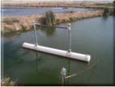
Water level control
