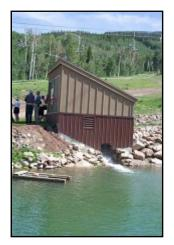
The plant's building houses a 115kW turbine attached to a 10-
