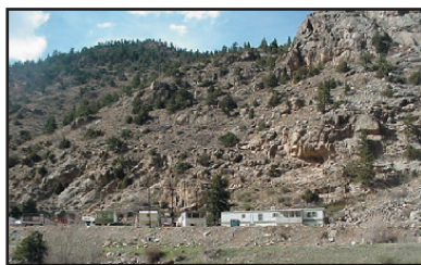
Rockfall Area Along I-70 Corridor Near Lawson, CO Photo by David C. Marlin
