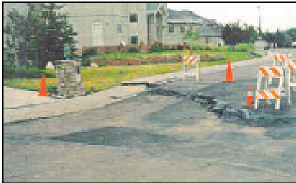
Scarp of the Green Mountain Landslide Photo by Colorado Geological Survey
