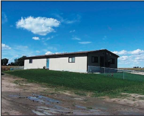
Building elevated in Morgan County Photo by CDEM
