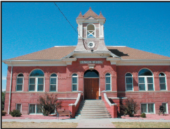
Floodproofed Historic Building Photo by Marilyn Gally
