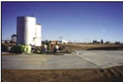
On farm mixing and loading pads can help protect workers and the environment.
