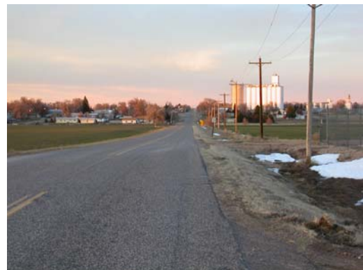
Looking North from the Substation Towards Haxtun
