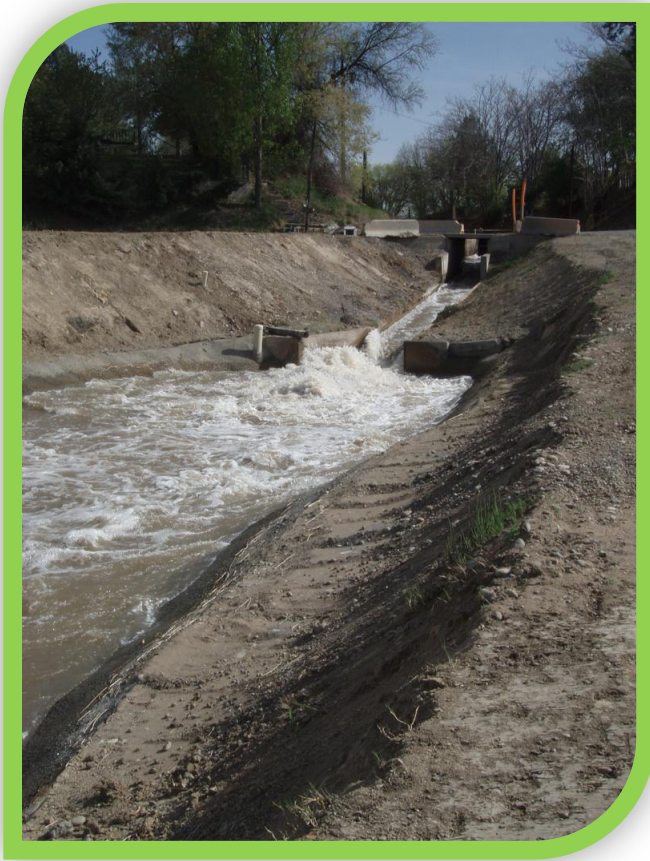
185 kW Dividers site photo
