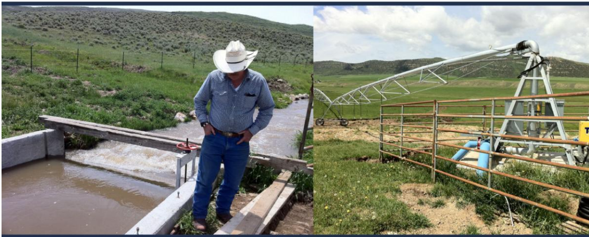
Rancher is utilizing a small hydro system in Colorado
