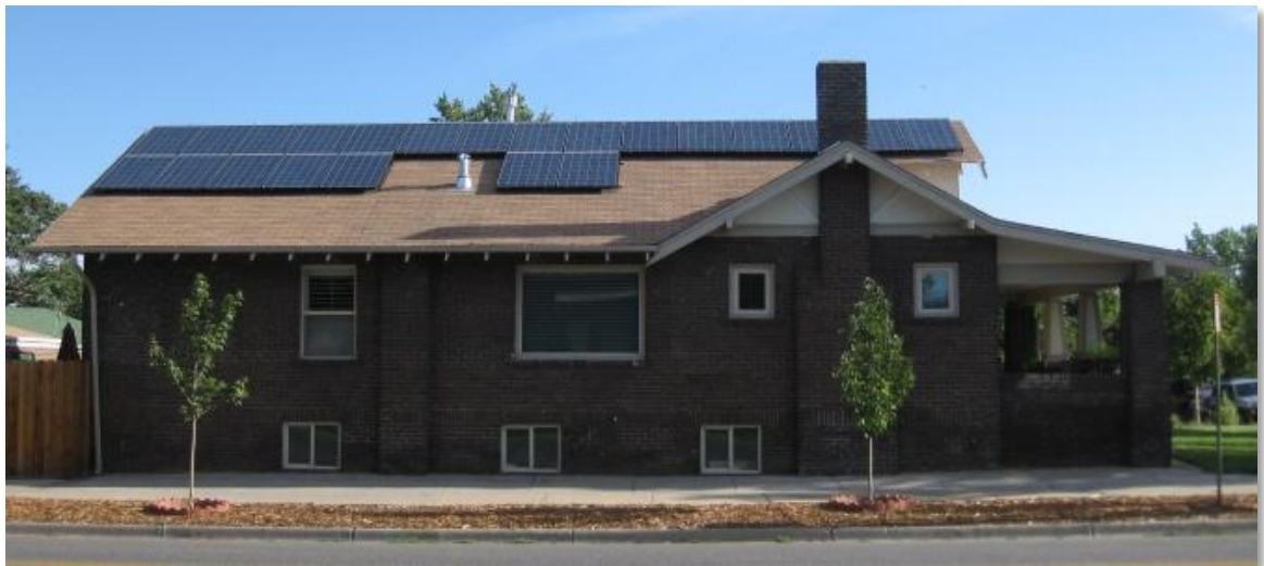
Figure 3. First Installation from the Solar Benefits Program
