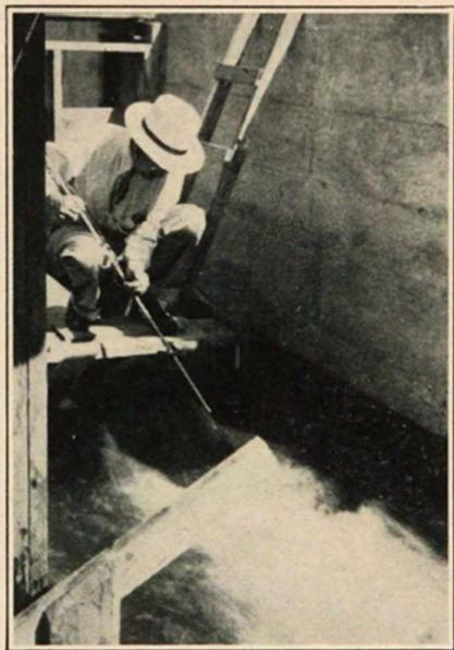
Figure 8—Hoff meter being held preparatory to starting measurement of pipe discharge.
