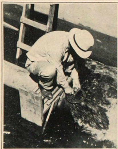
Figure 15—Measuring angle of spiral flow with protractor.
