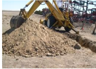
Soil excavation for tower foundation design.
