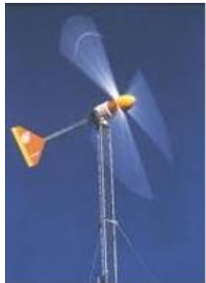
10 kW turbine on guyed lattice tower
