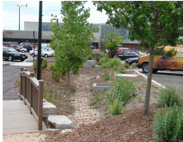
Aurora parking lot runoff directed to a grass swale through a slotted curb (left). Bioswale in a Colorado Springs parking lot (right). (Photos Courtesy of Michelle Delaria, CASFM photo database, http://www.casfm.org/stormwater_committee/ ).
