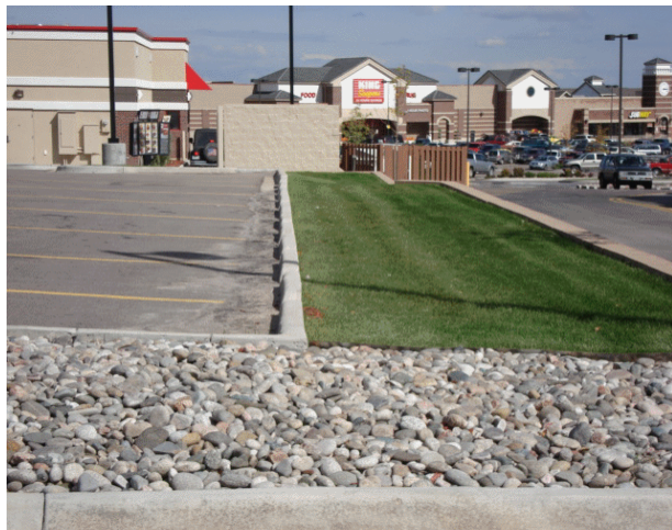
Aurora parking lot runoff directed to a grass swale through a slotted curb (left). Bioswale in a Colorado Springs parking lot (right). (Photos Courtesy of Michelle Delaria, CASFM photo database, http://www.casfm.org/stormwater_committee/ ).
