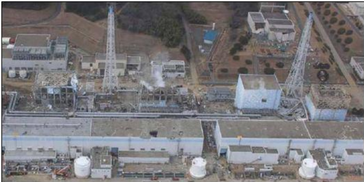
Figure IX-41 Fukushima Dai-ichi Nuclear Power Plant Units 1 – 4 after explosions
