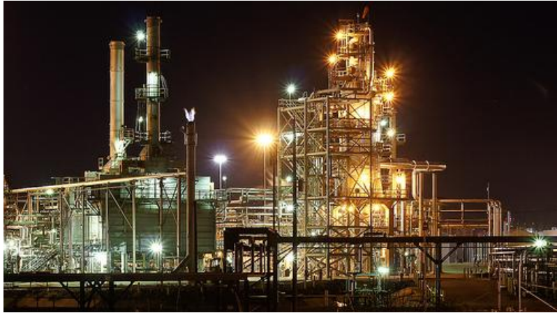
The Suncor Refinery in Commerce City, CO
