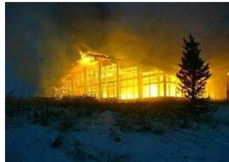
Arson has been a favored method of physical attack by environmental extremist groups. In 1999, individuals affiliated with the Earth Liberation Front burned several buildings at the Colorado's Vail Ski Resort. The Vail arson caused over $12 million in damage. Upon apprehension, the perpetrators of the Vail arson later pled guilty to a campaign of environmentally-motivated arsons from 1996-2001, totaling over $20 million dollars in damage.
