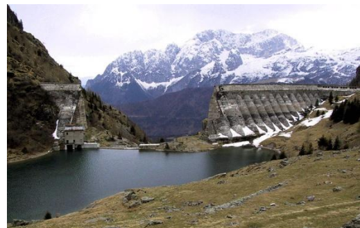
Remains of the Gleno Dam, which failed due to faulty engineering in 1923.
