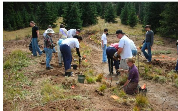
The Pikes Peak Watershed Erosion Control and Restoration Project: removing over 270 cubic yards of sediment from the Glen Cove wetland area. Image from the Rocky Mountain Field Institute
