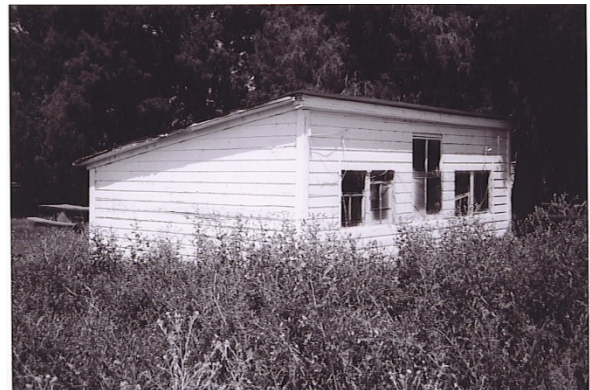
Building 8: chicken brooder house, front elevation, view to northeast
