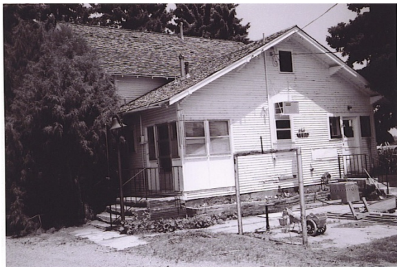
Main House: rear elevation, view to northeast
