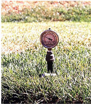
Pressure gauge on a fixed spray head
