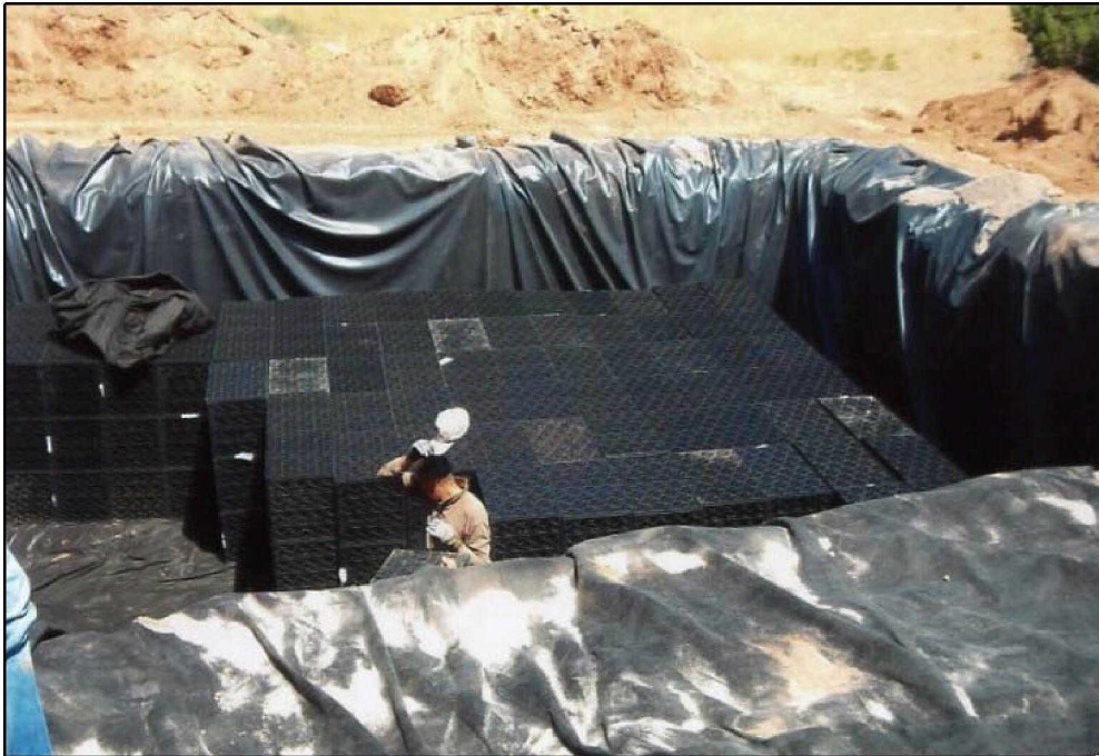
Figure 13. Cistern Installation
