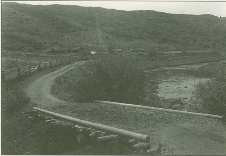
View of the ranch house, December, 1967, Jackson County, Colorado.
