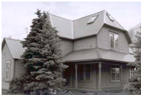
CF&I Superintendent's House
