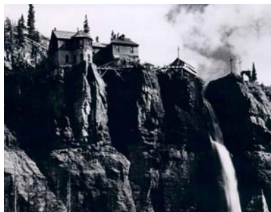
Smuggler-Union Hydroelectric Power Plant/Bridal Veil Powerhouse
