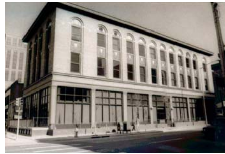
General Electric Building
