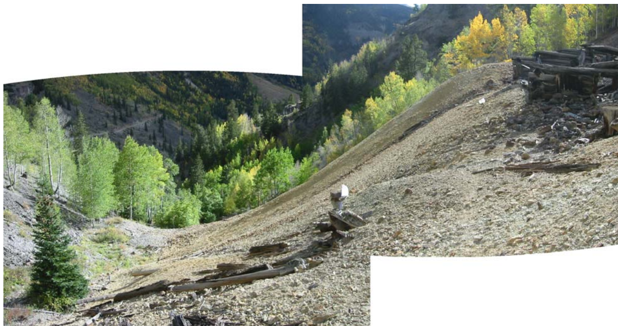
Figure 43. Lellie Mine (Site #54) and adjacent drainage
