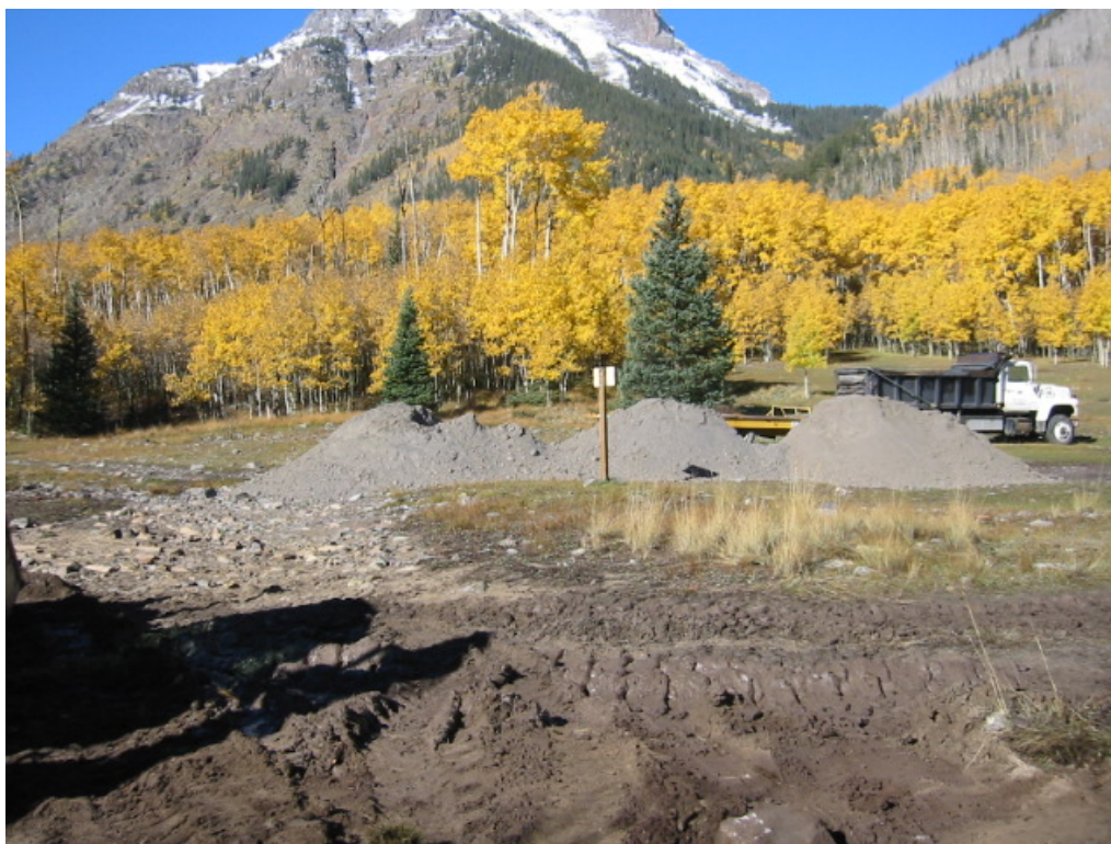
Figure 33. Hanna Mill Tailings during reclamation in September 2005
