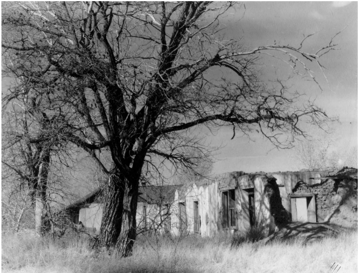
Figure 11. Lafayette Head’s home in Conejos was deteriorating rapidly in 1969, shortly before it was razed. “Fort Head” was also a trading post and the Southern Ute Indian Agency from 1861 to 1868 (see Simmons 1999:90, 92). Photo by Ruth Marie Colville, OAHN site files, 5CN501.
