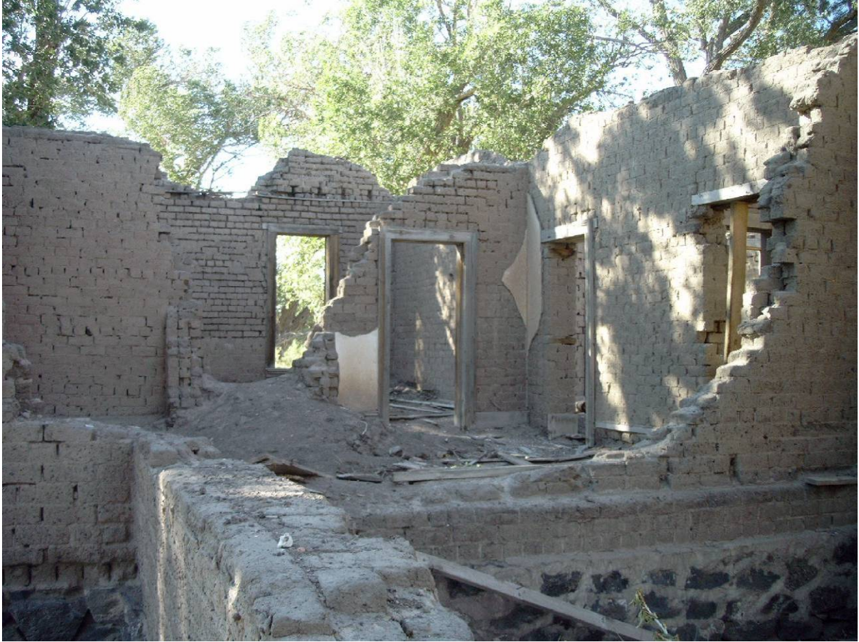
Figure 14. The McIntire Ranch home is an example of Territorial Adobe style architecture, with three-brick-thick walls made of adobe mud.
