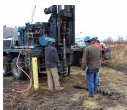
Drilling a monitoring well (above) and the completed well (below).
