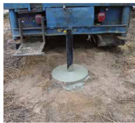
Drilling a monitoring well (above) and the completed well (below).
