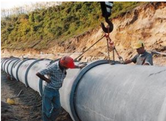
Figure 35: Concrete Penstock with Spun Rubber Ring Joints
