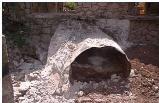
Figure 32: Deteriorated Penstock
