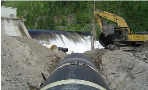
Figure 39: HDPE Penstock
