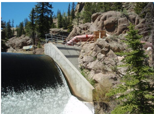
Figure 6: Humphreys Hydro Siphon Intake (Upper Right)
