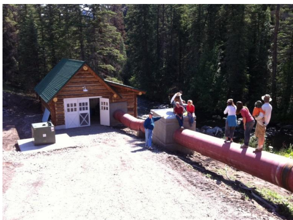
Figure 5: Humphreys Hydro Powerhouse
