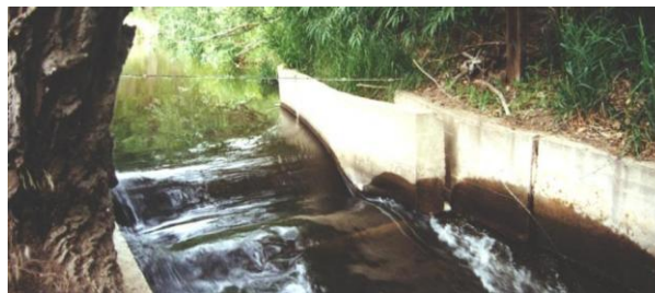
Figure 18: Parshall Flume in Box Elder Ditch, Cache la Poudre
