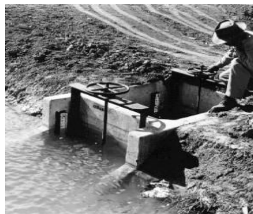
Figure 22: Constant Head Orifice Turnout
