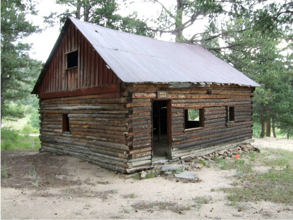
Figure 16. View northeast at the Dutch Louie cabin, site 5LR11798, showing the doorway in the south elevation, windows, and rock foundation.
