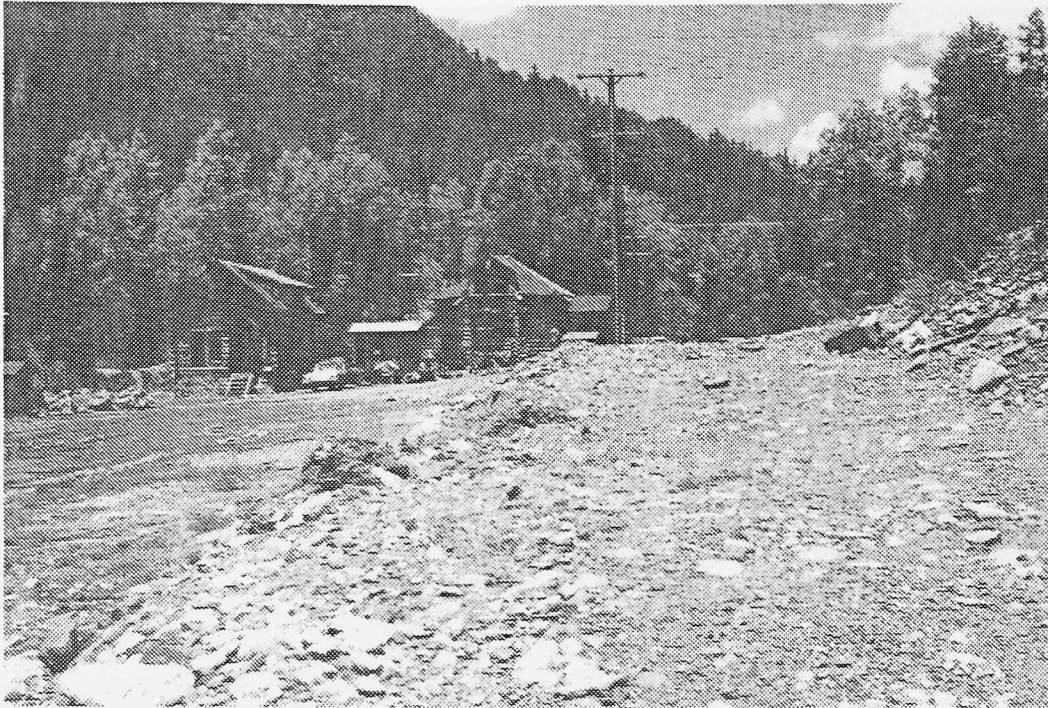
Figure 6. Looking north toward the most seriously affected properties. The main haulage adit is in the trees on the right of the picture.
