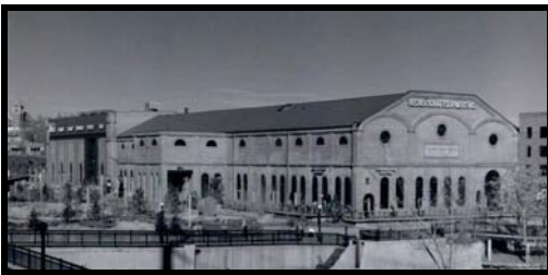
Denver Tramway Powerhouse, 2001
