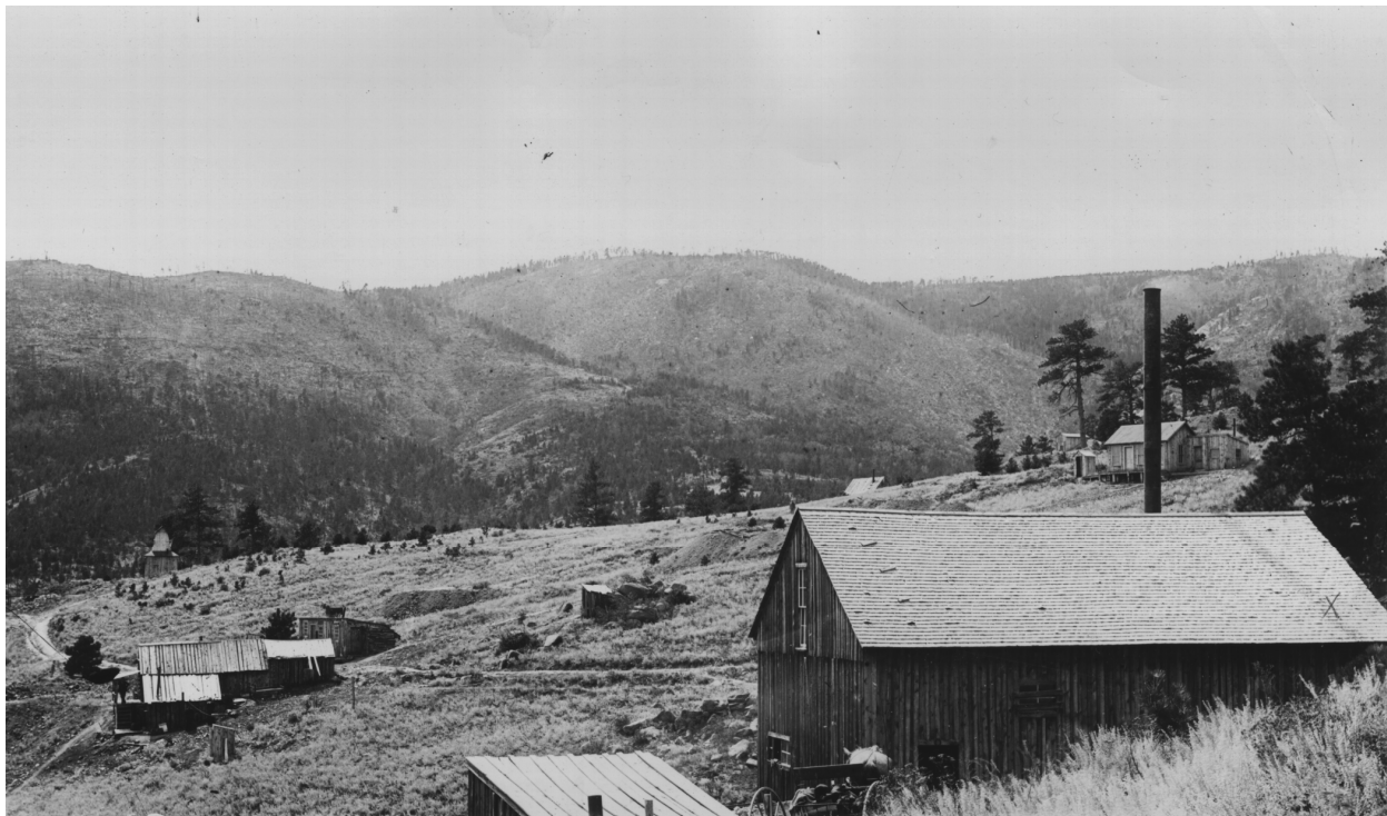
Figure E 4.10.2. The Magnolia Mining District was the scene of a frenetic rush during the late 1870s. This south view depicts the principal concentration of mines in 1876 or 1877, when they were in states of development. Many failed and were abandoned in primitive states. The town, which remained small, extends right and out of view. Source: Boulder Carnegie Library, 219-8-66.
