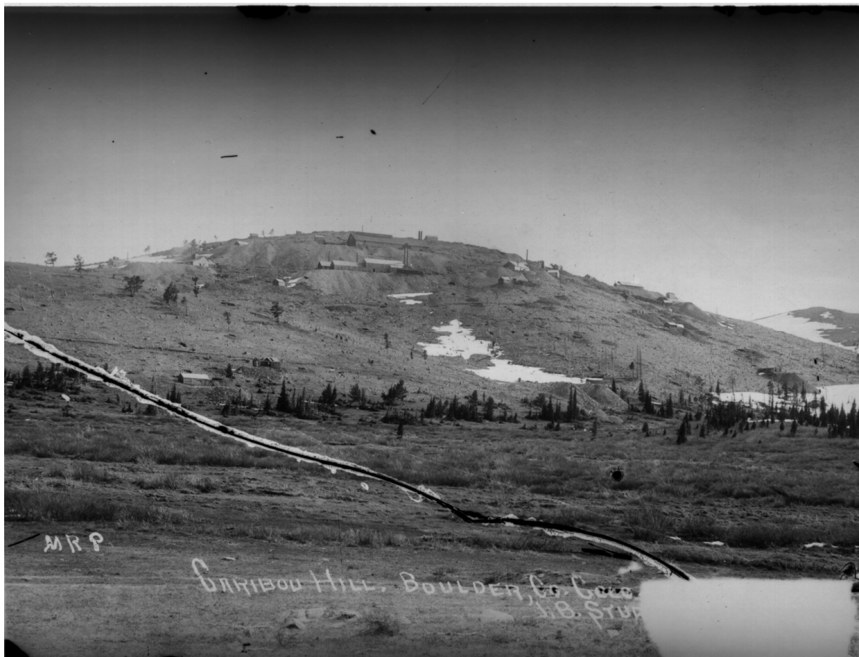
Figure E 4.3.2. Caribou Hill was the economic and industrial center of the Grand Island Mining District as it existed around 1880. The long, dark shaft house immediately below the hilltop belonged to the Caribou Mine, and the waste rock dumps at the hill base right of center mark the Seven-Thirty Tunnel. The town of Caribou is left and out of view. Source: Boulder Carnegie Library, 219-2-9.
