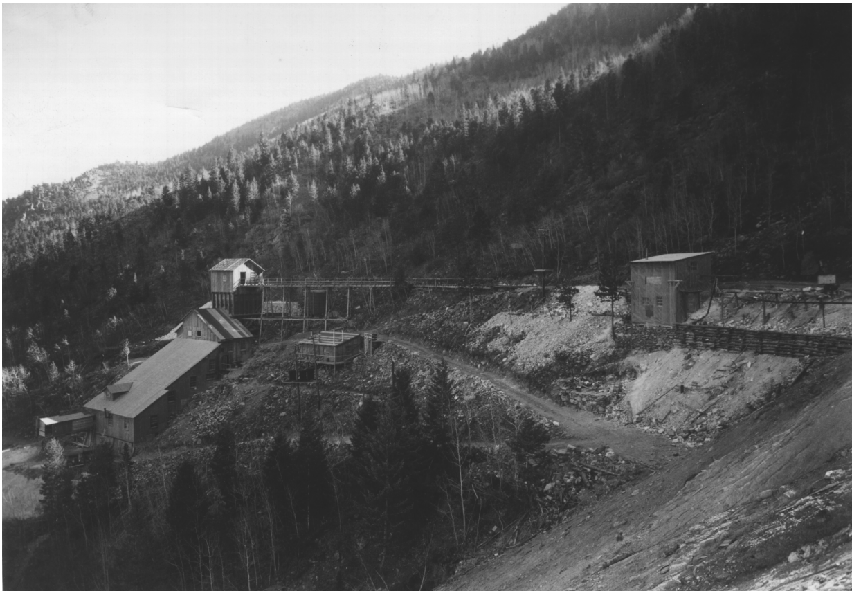
Figure E 4.6.6. Around 1934, Slide Mines built a new mill at the mouth of the Corning Tunnel. The operation was one of Gold Hill's most profitable and a significant employer, both of which were important in the climate of the Great Depression. The tunnel is right and out of view. Source: Boulder Carnegie Library, 219-8-9b.
