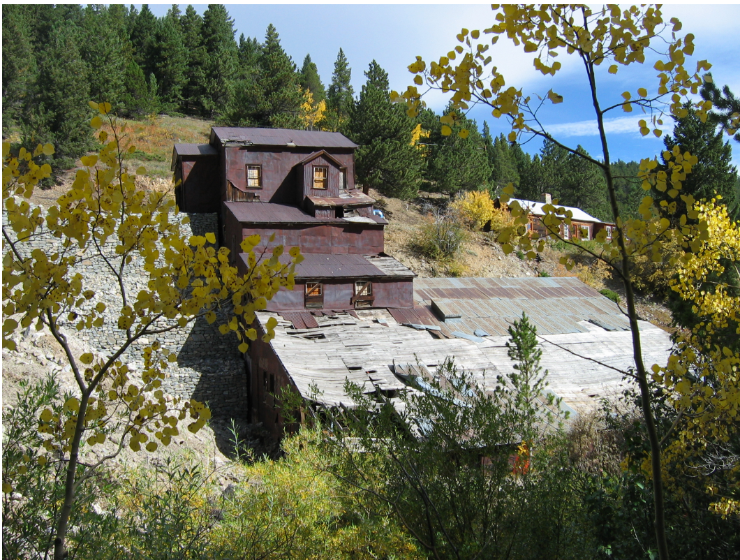
Figure E 4.3.4. Today's Cardinal Mill, formerly known as the Boulder County and the Midget, has changed little since it was built during the 1890s. The Boulder County Tunnel is left and out view. Source: Carol Beam.
