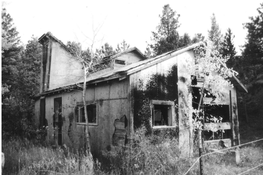
Figure E 5.2.39. After shaft houses were outlawed during the 1910s, mining companies erected hoist houses to enclose critical facilities. The Blue Jay Mine's hoist house, near Jamestown, is a typical example. The left roofline features an angled cupola for the hoist cable, which ascended to a headframe left and out of view. Source: Author.
