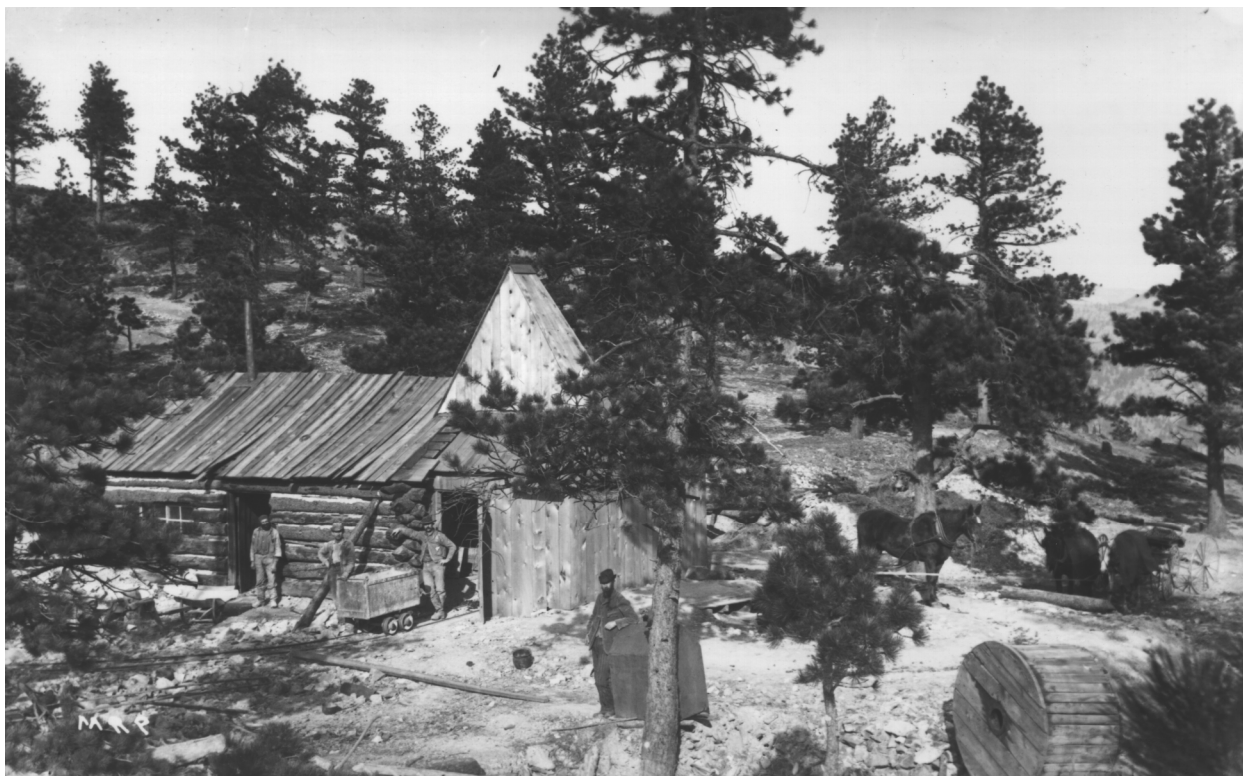
Figure E 4.7.2. In 1874, shortly after discovery, the American Mine was primitive and typical of many frontier shaft operations. A hoist and shop occupied the log building at left, and a headframe stood under the tall peak. One of the individuals is discoverer Hiram Fullen. Source: Boulder Carnegie Library, 219-1-8.
