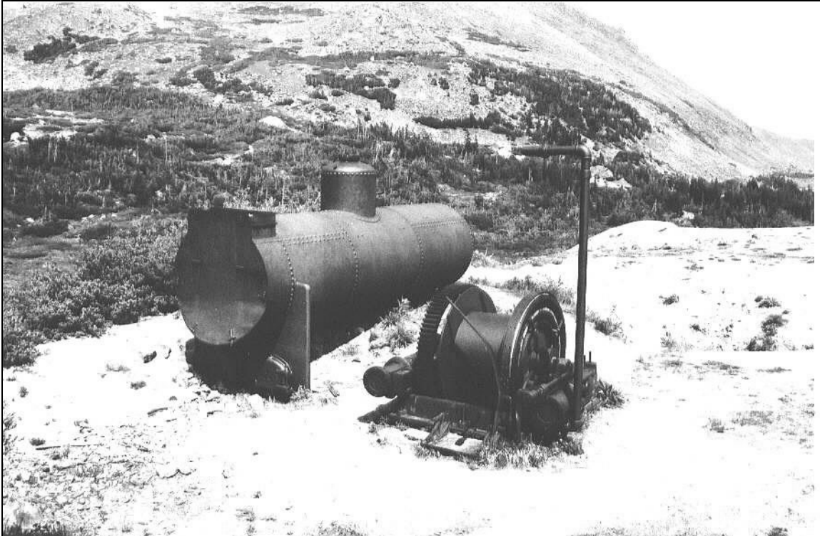
Figure F 4.1. While the Fourth of July Mine was never profitable, it was equipped with a production-class surface plant. The shaft house is long gone, but the hoist and boiler currently remain and can be accessed via the Fourth of July Trail west of Caribou. Source: Author.
