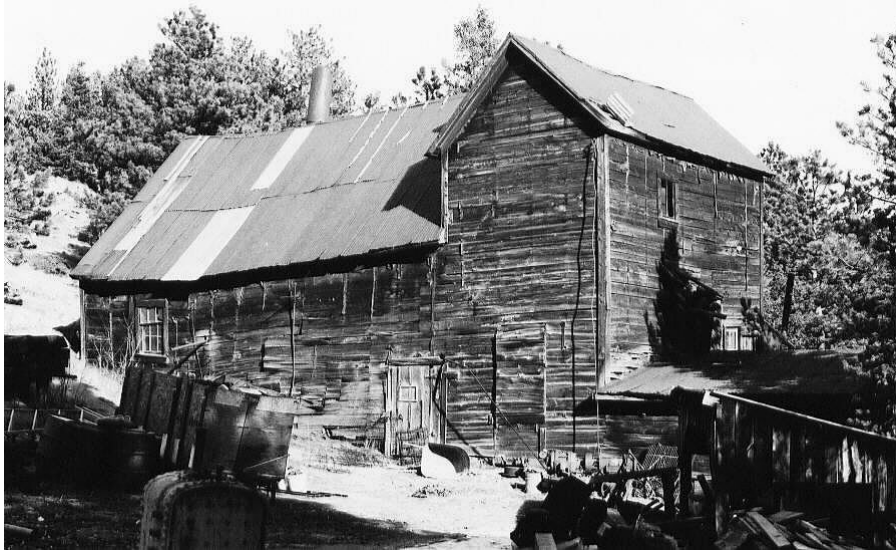
Figure E 5.2.38. Most of Boulder County's mining companies erected shaft houses similar to this modest one at the Snowbound Mine, pictured above. The building is well-built and is based on a balloon frame. Common at one time, shaft houses are now important and rare structures. Source: Author.
