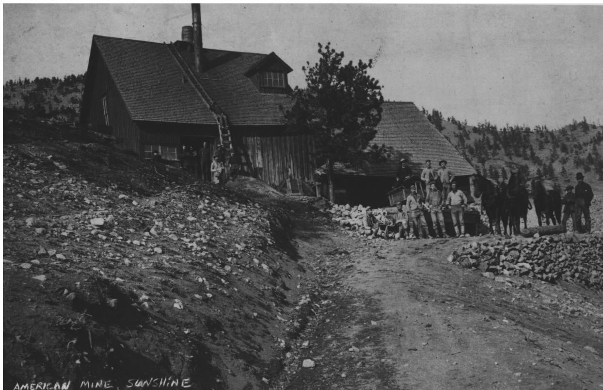
Figure E 4.7.3. New York City capitalist Hiram Hitchcock purchased the American Mine in 1876, invested in a substantial steam plant, and sank the shaft deeper. Hitchcock was amply rewarded for his expense, and the American became one of Sunshine's most important mines. The structure at left enclosed the shaft and hoisting system, and the shed at right was an ore sorting house. Source: Boulder Carnegie Library, 219-1-9.
