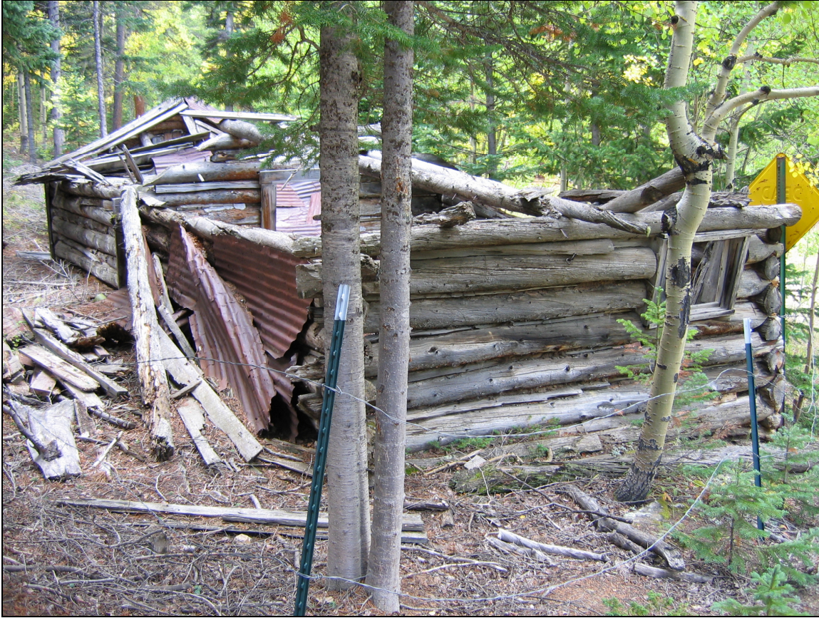
Figure F 8.2. When intact, this structure in Boulder County was a typical log cabin, but it has decayed into what is currently termed a cabin remnant . These types of cabins were a universal form of housing at mines and in towns. Source: Carol Beam.
