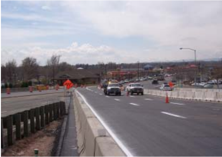
The temporary alignment on Wadsworth Boulevard near Grandview Avenue (Project #2).
