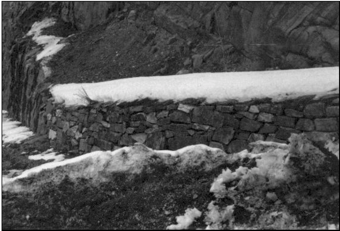
Plate 12. Dry-laid stone wall south of Ouray Tunnel on US 550.
