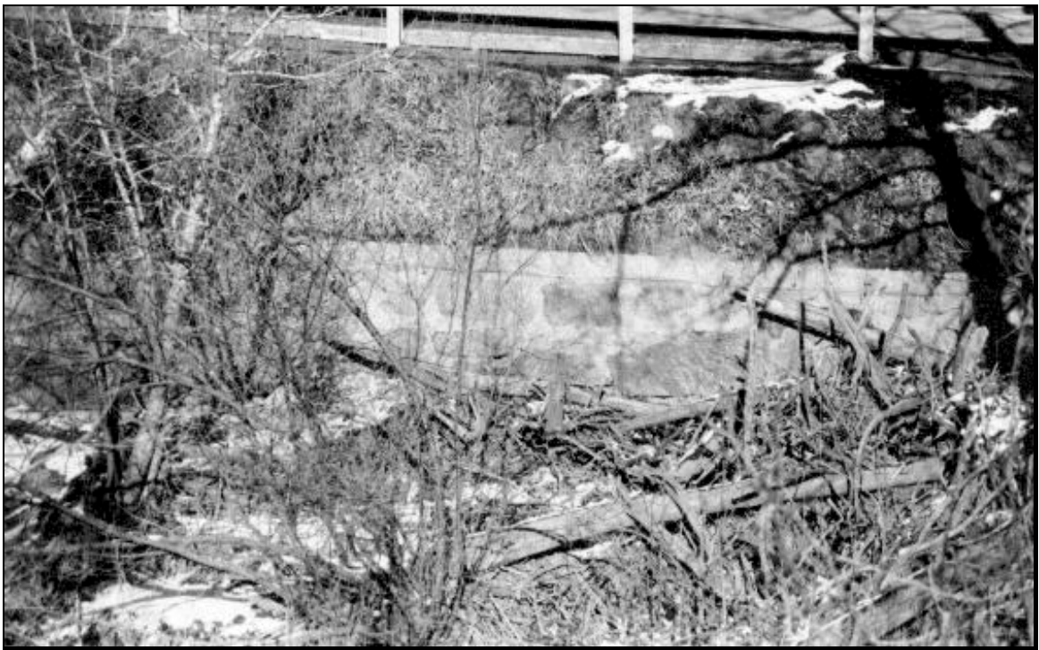
Plate 35. Cement rubble masonry wall along Fountain Creek on US 24.
