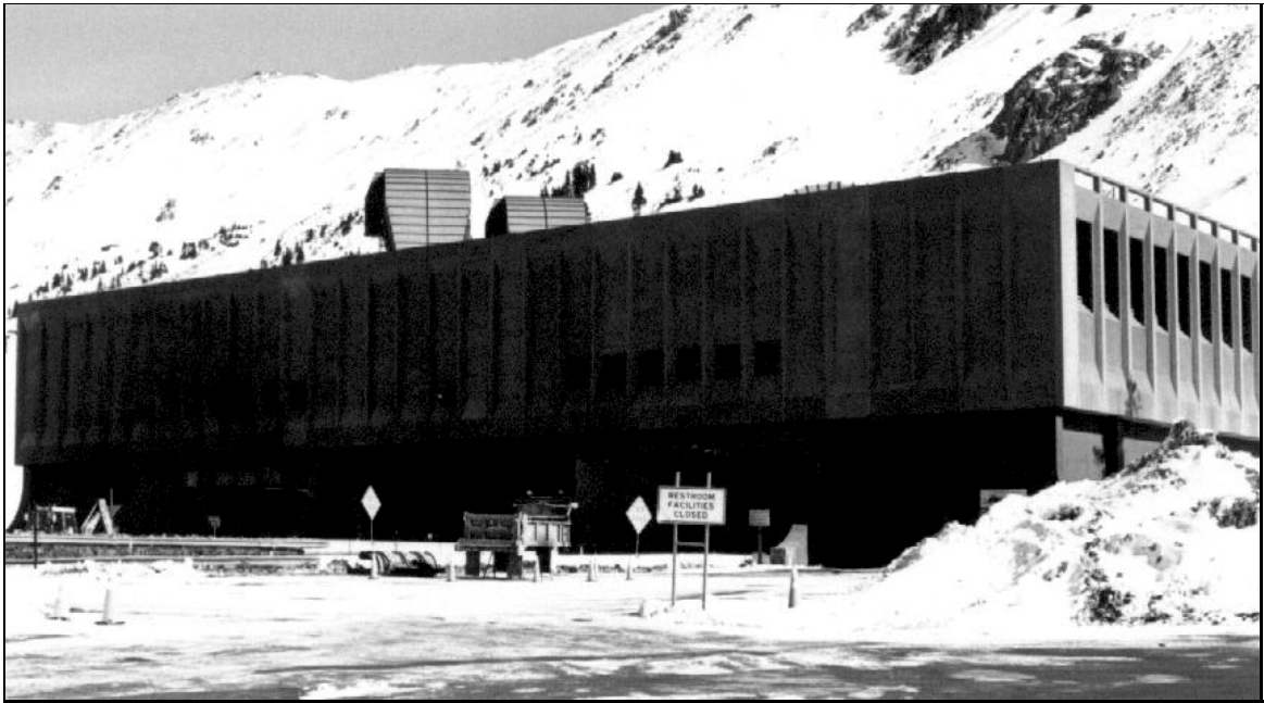
Plate 33. Eastbound bore (named for Colorado Governor Edwin C. Johnson) of the Eisenhower Tunnel.
