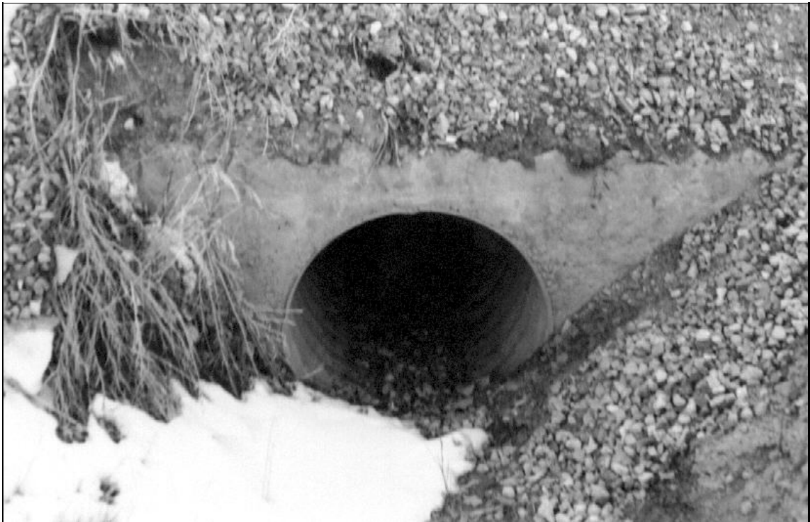
Plate 30. West view of concrete culvert beneath old alignment of SH 13.
