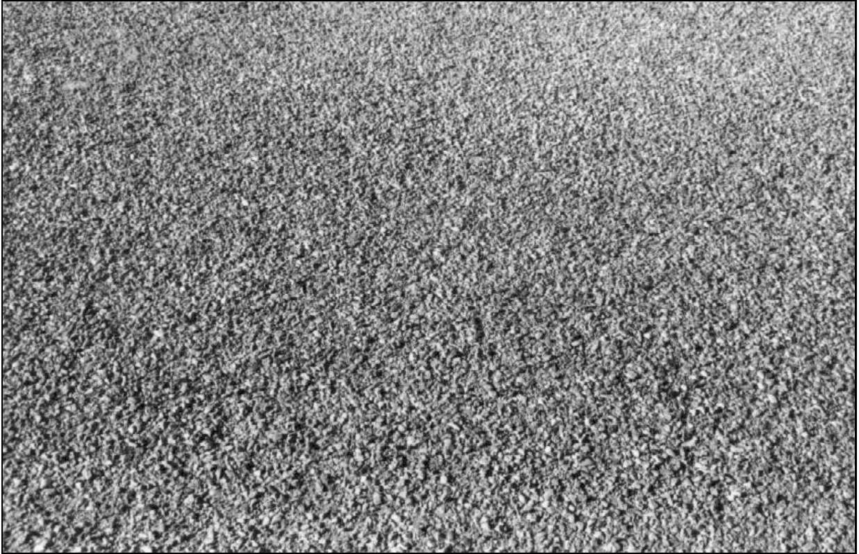
Plate 24. Large chunks of aggregate on old US 85; approximately 500 feet west of I-25.
