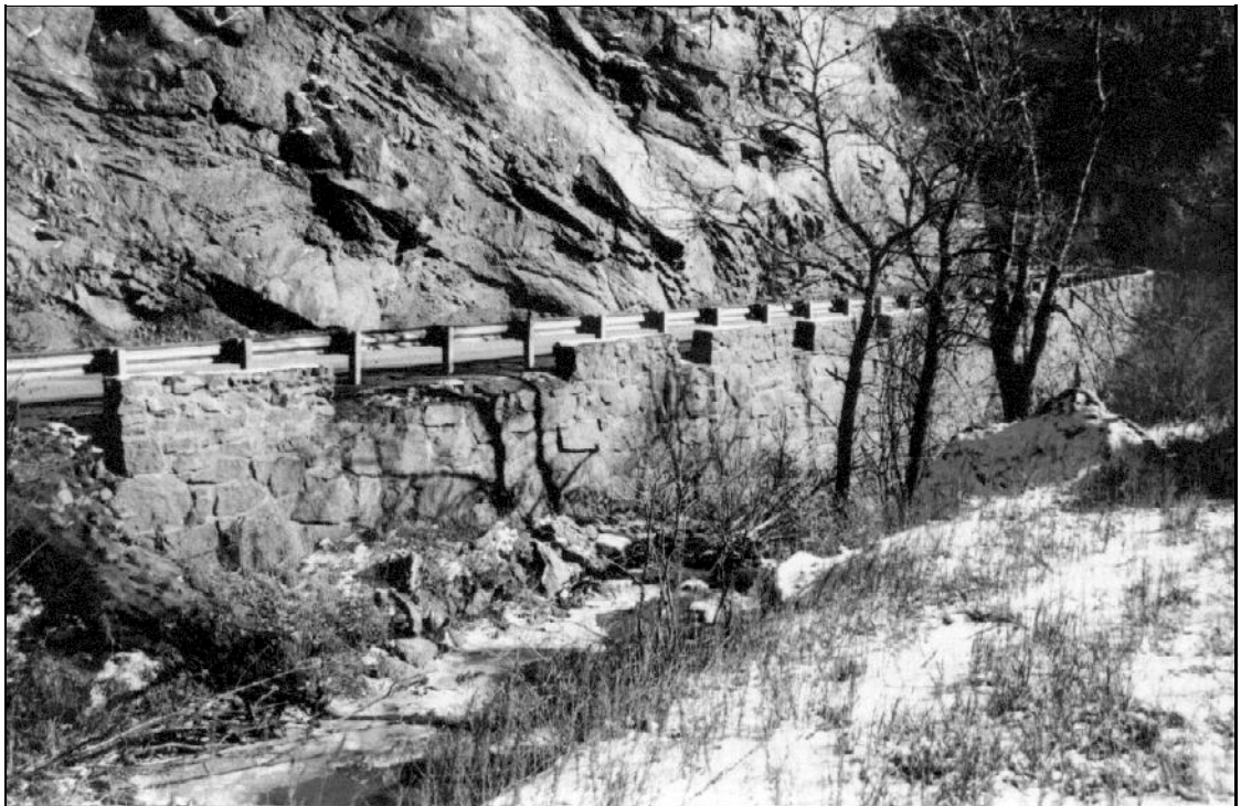
Plate 37. Stonework along Fountain Creek. View from eastside of US 24.
