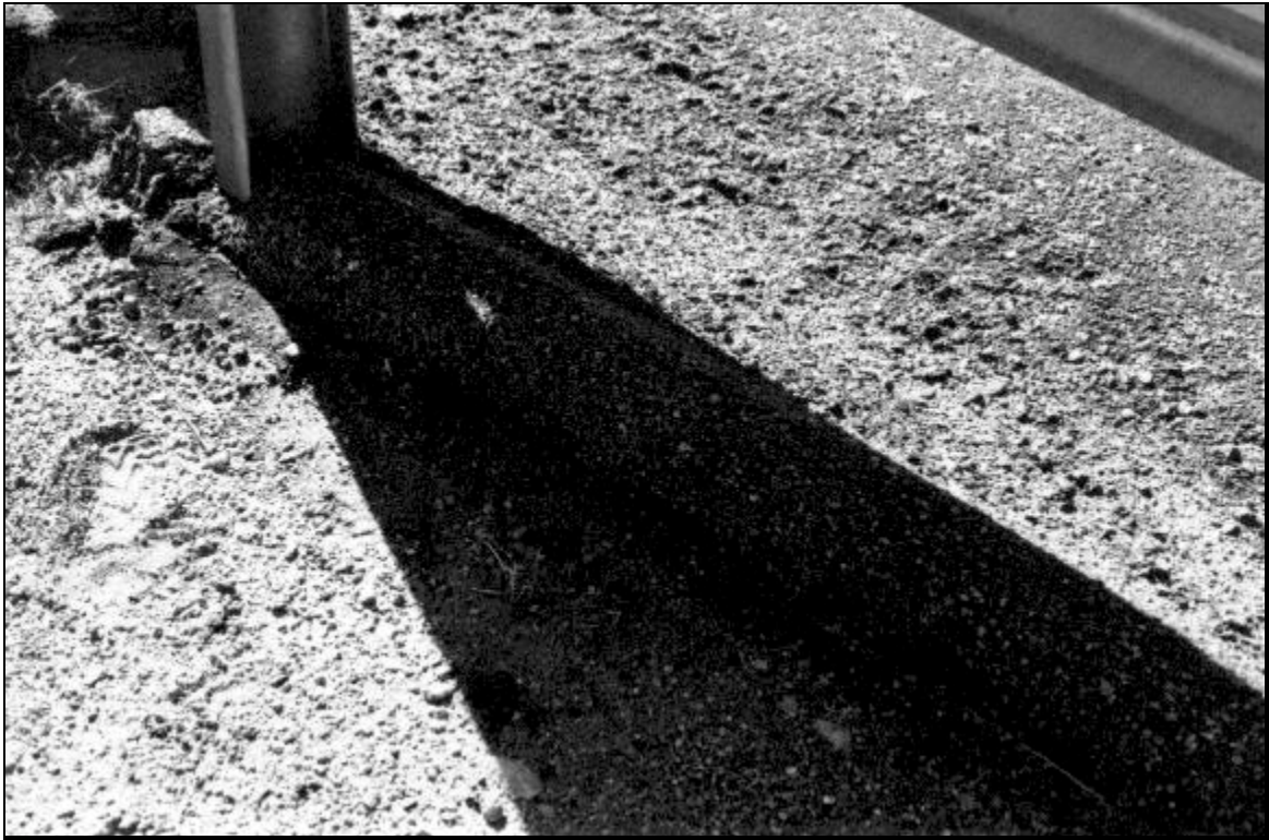
Plate 22. Asphalt mountable curbing inside guardrail on US 6.
