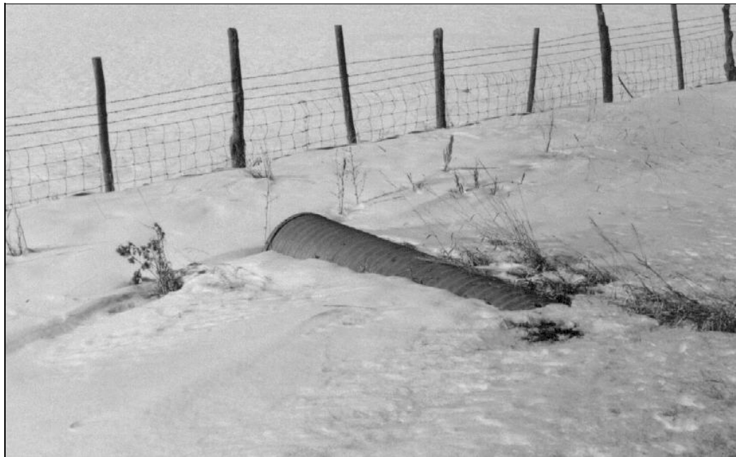
Plate 32. Corrugated metal culvert viewed from the west side of SH 13.
