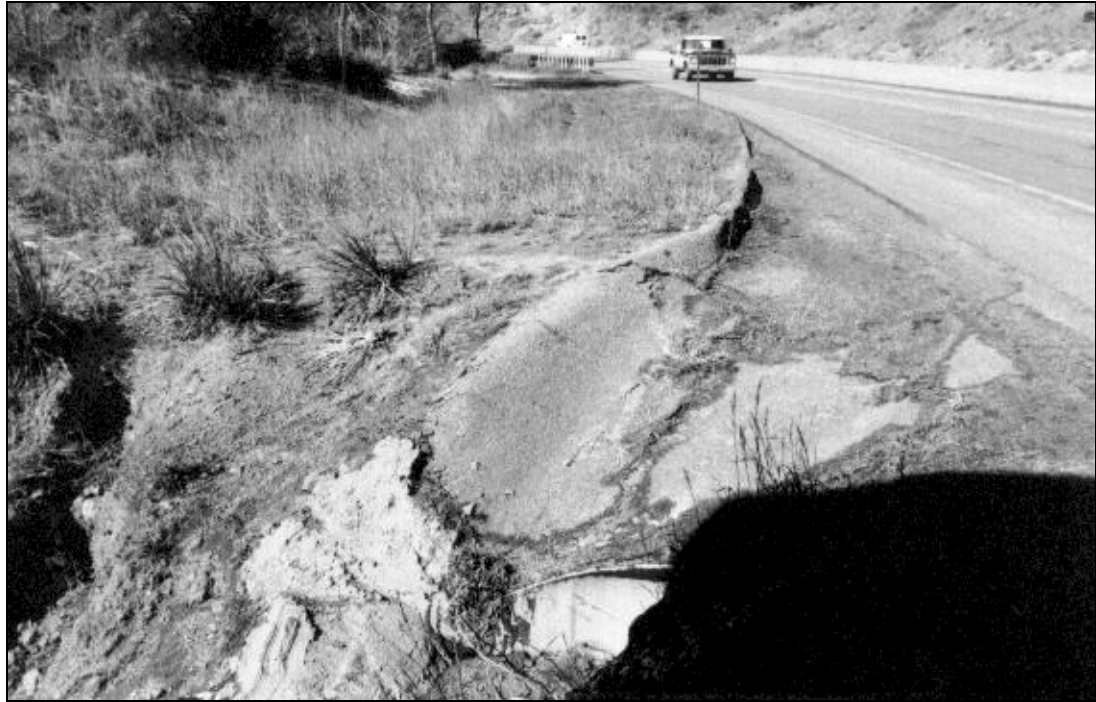
Plate 38. Curbing placed by PWA crews during the 1930s on US 24 west of Manitou Springs. Materials included a mixture of red rock and asphalt.
