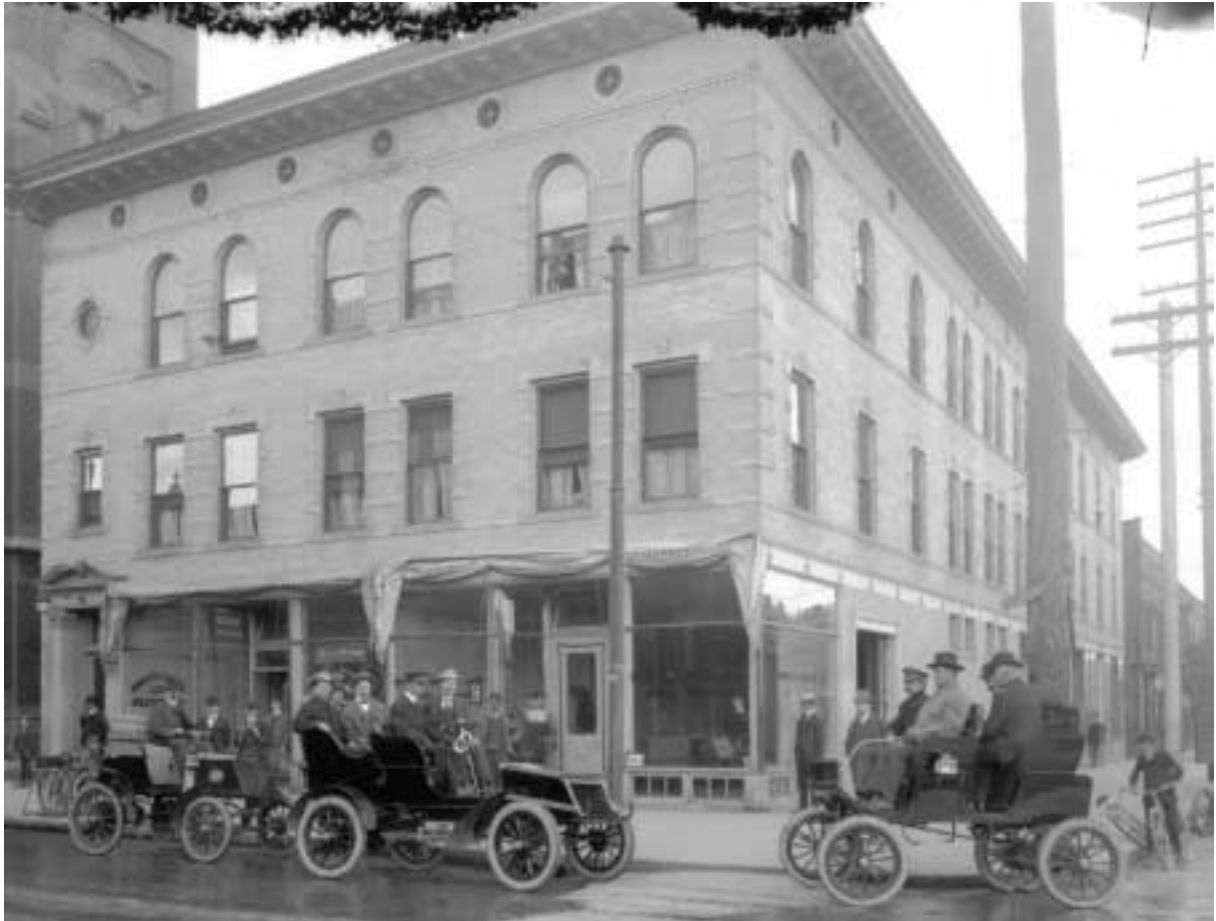
Plate 3. Bumper-to-bumper traffic held a different meaning on the streets of Denver at the turn of the 20 th century. These proud horseless carriage owners met at the corner of 18 th and Stout in front of the Colorado Winton Motor Carriage Company. Source: Denver Public Library, Western History Department. ©1995-2002 Denver Public Library.
