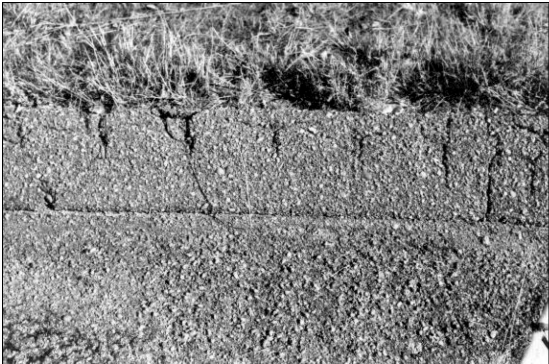
Plate 23. View east of curbing leading to drainpipe near South Platte River on US 6.
