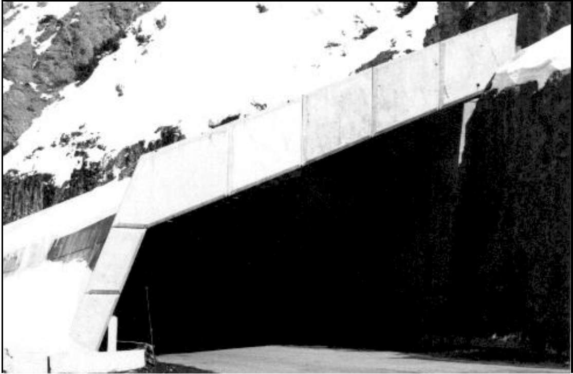
Plate 11. Northeast view of Riverside Slide, a block and concrete tunnel.
