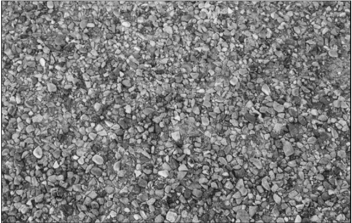
Plate 29. Bituminous concrete on old alignment of SH 13 in Rifle.
