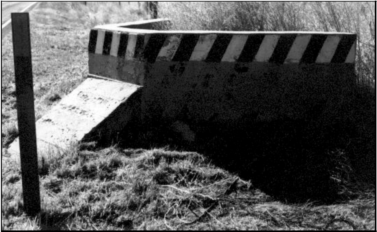
Plate 20. Raised culvert on north side of US 6 (c. 1925). Culvert stands 2'8" high.
