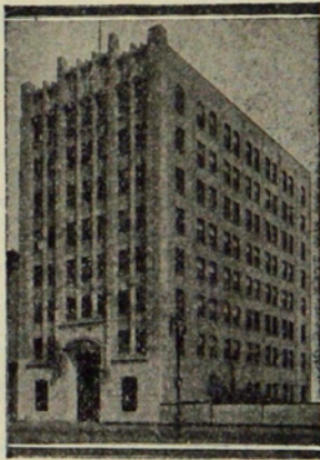
New Wheat Pool Office Building at Winnipeg, Man., Canada
