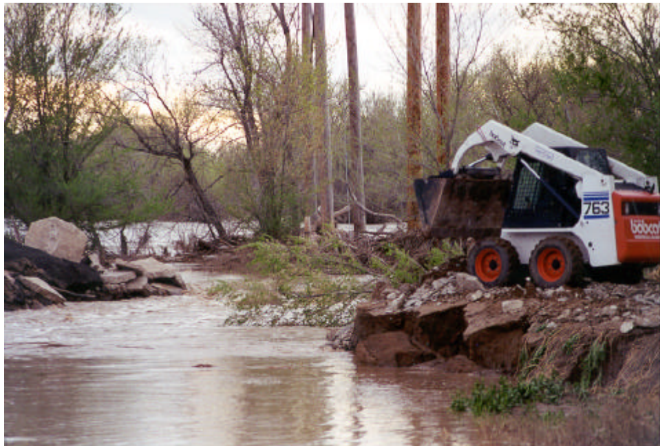
Repairing a levee break in North La Junta. May 3, 1999
