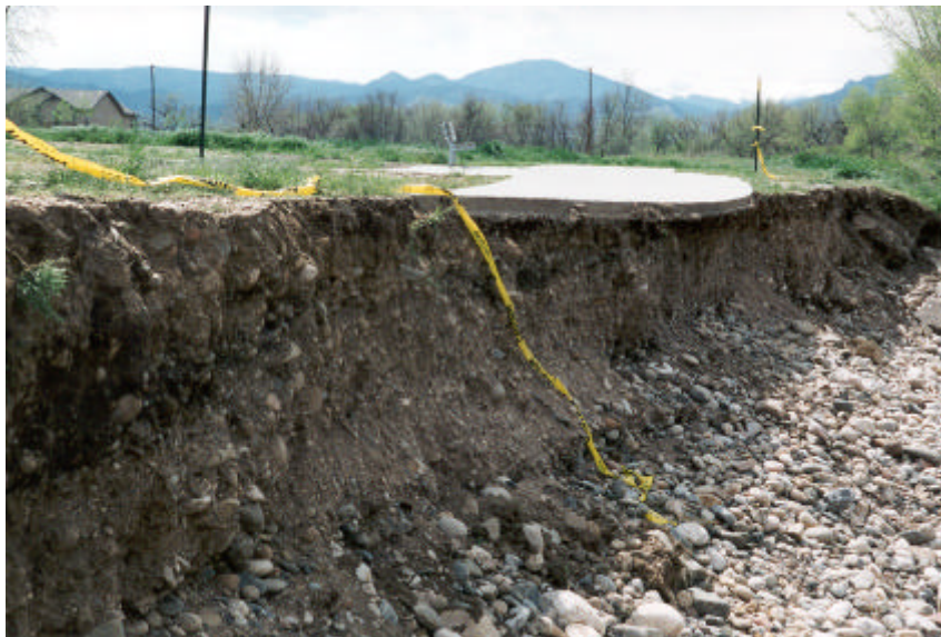
Bike path washout near Taft Avenue along the Big Thompson River in Loveland.
