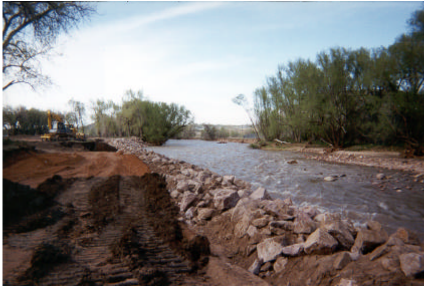
Emergency work complete on Fountain Creek bank south of Circle Drive.
