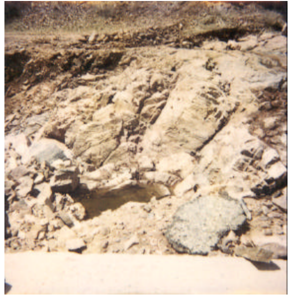
Damage to County Road 67, Phantom Canyon.
