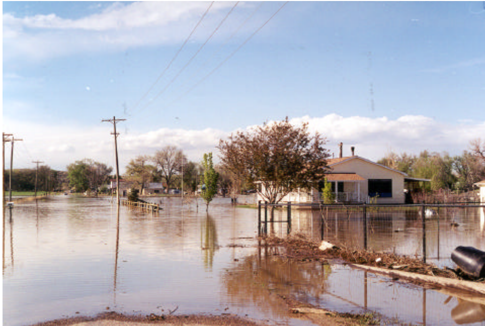
Floodwaters in North La Junta. May 4, 1999
