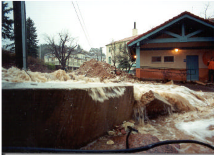
Floodwaters break the retaining wall at Soda Springs Park in Manitou Springs.
