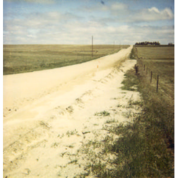
Sediment deposited along CR 149 at the intersection with CR 66.
