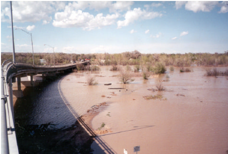
Arkansas River at Main Street bridge looking north.
