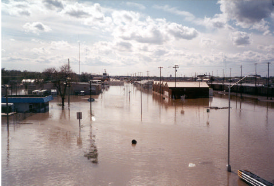
Looking west at flooded businesses in La Junta near Bradish and Highway 50. May 4, 1999
