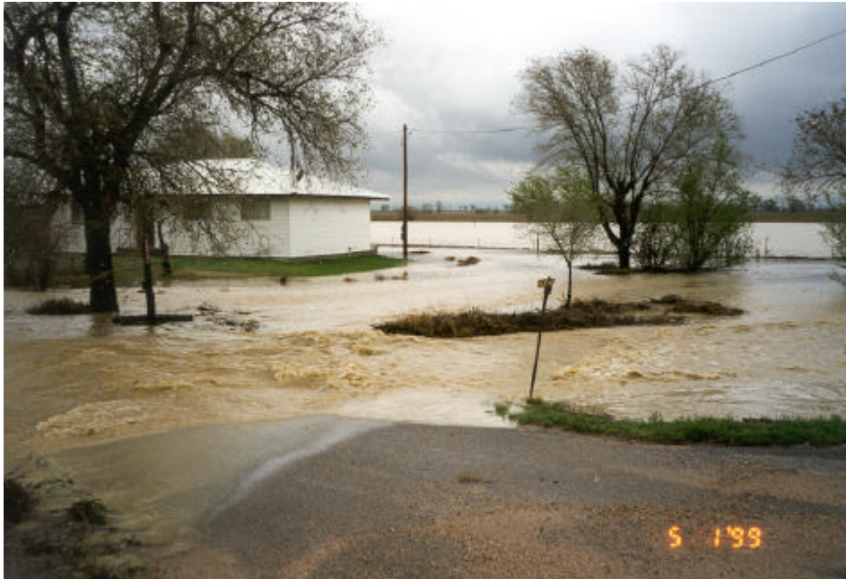
Flood flows and a home on Highway 96.
