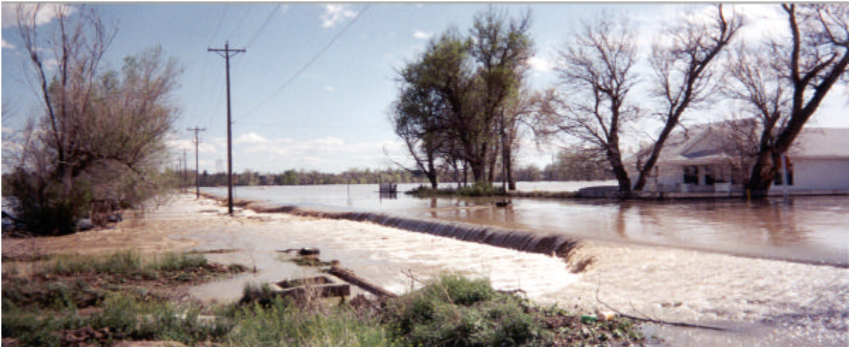
Overtopping and erosion of road in North La Junta.
