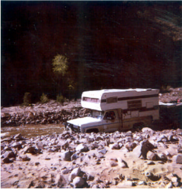
Damage to County Road 67, Phantom Canyon.
