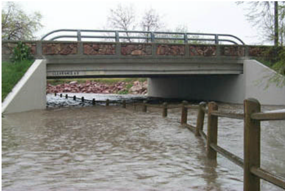
High water in Spring Creek at Riverside Bridge in Fort Collins.
