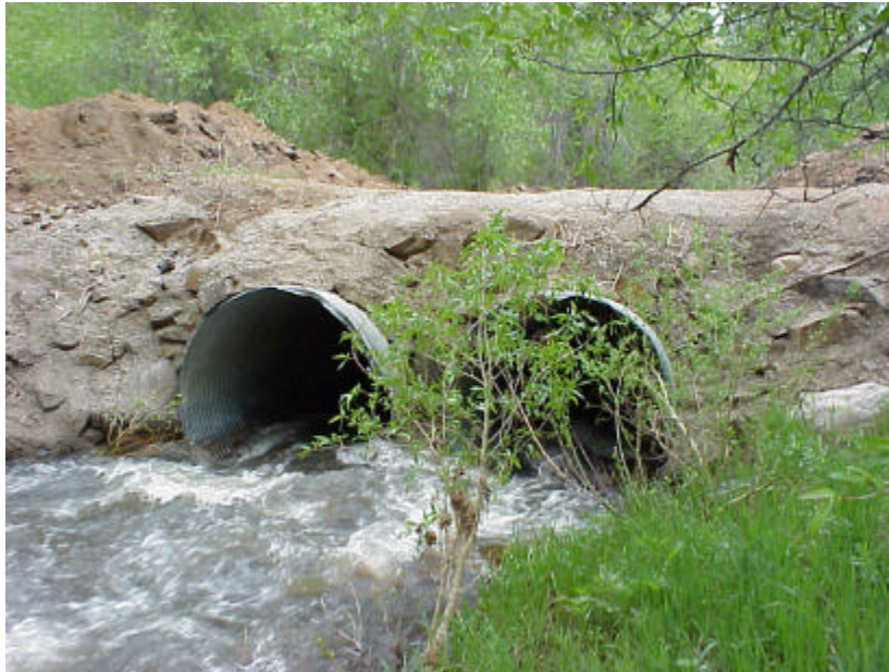
Completed repairs to County Road 389 culvert crossing.
