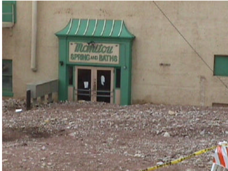
Debris fan at Manitou Springs bath house.
