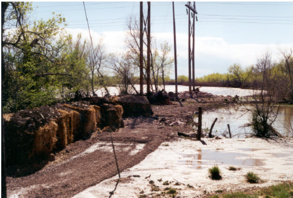
Temporary dike in North La Junta. May 5, 1999
