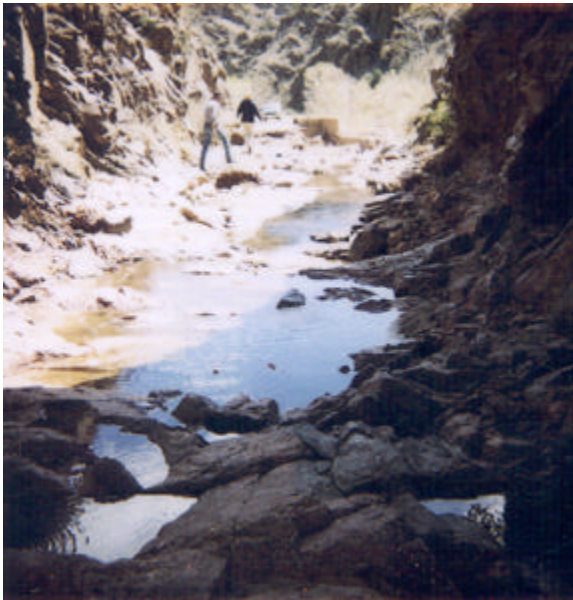
Damage to County Road 67, Phantom Canyon.
