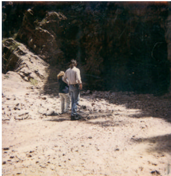
Damage to County Road 67, Phantom Canyon.
