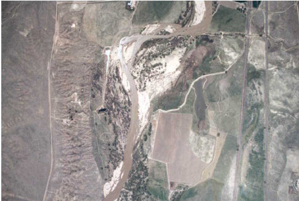
Erosion along Fountain Creek north of the Totten residence.
