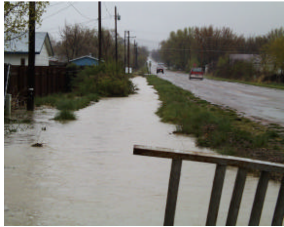
Channel on west side of Orchard Avenue between Central and Pear in Cañon City. Channel carries water from the Orchard Avenue Detention Basin to Pear Avenue.
