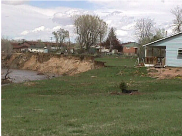
Fountain Creek erosion threatening homes in the City of Fountain.
