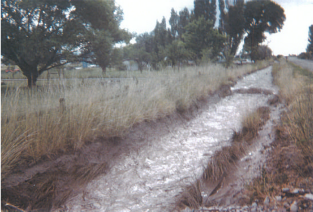
Bosley Wash at 3445 F \frac{3}{4} Road (1999 storm event).
