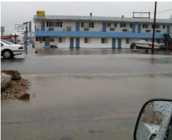
Northwest corner of Royal Gorge Boulevard (Highway 50) and 13 th in Cañon City. This is typical flooding at this location even after moderate rainfall.
