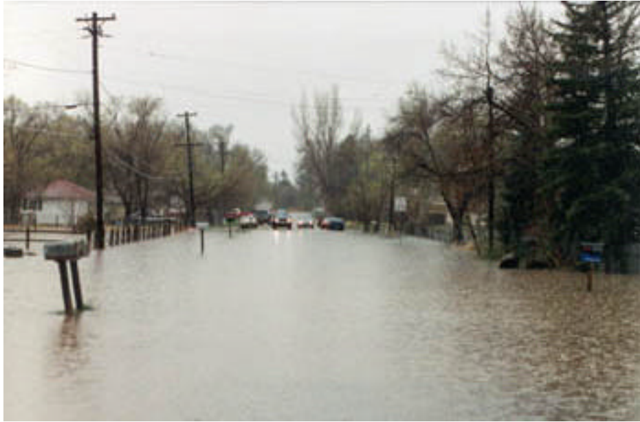
Flooding at Hollywood and Cherry Streets in Larimer County.
