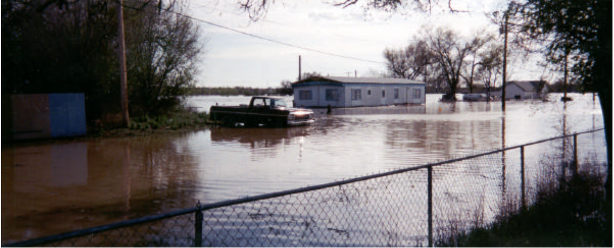
North La Junta trailer elevated approximately 7 ft to 100-year flood plain elevation.
