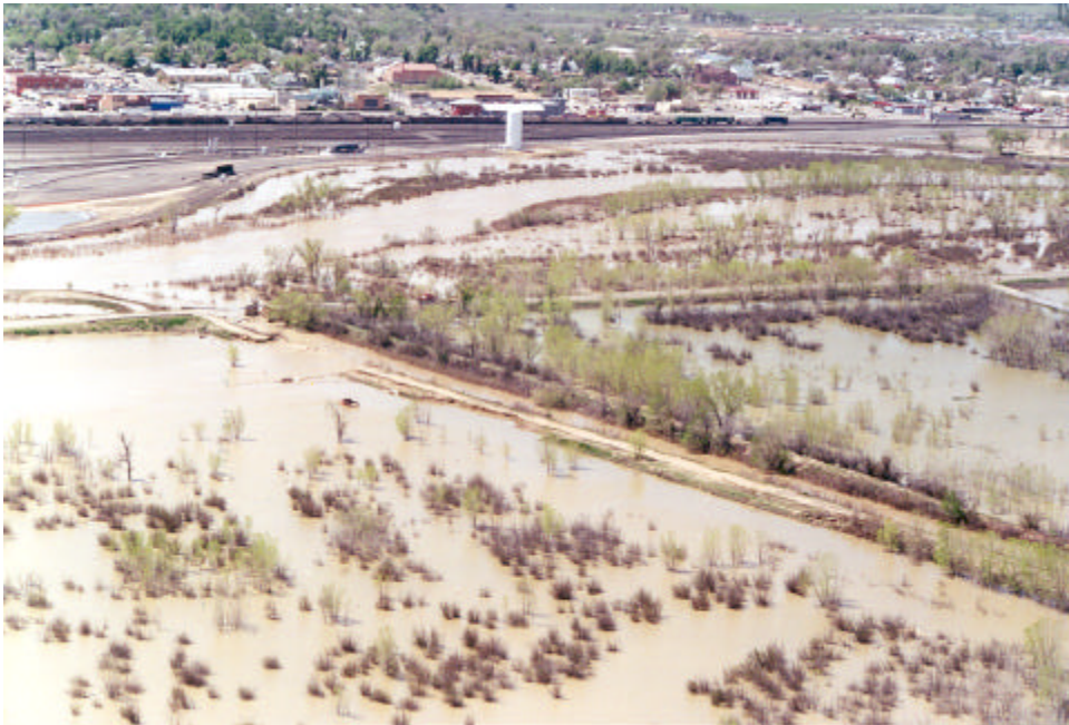
Break in the Fort Lyon Sluice #2 and a washout on Dike Road in North La Junta. May 3, 1999
