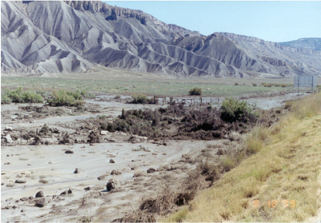
Bosley Wash at I-70 Culvert Inlet (August 11, 1999).
