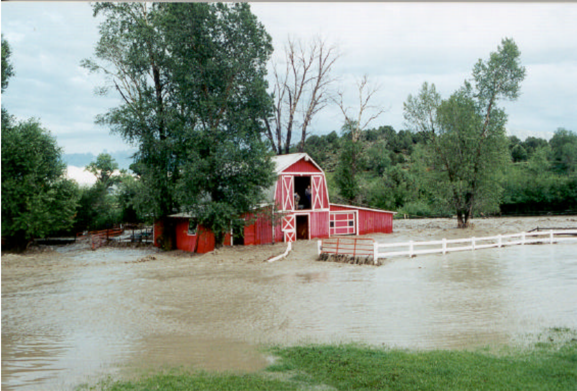
Flooding along Dallas Creek near County Roads 5 and 24. Note high-water marks on lower level walls.
