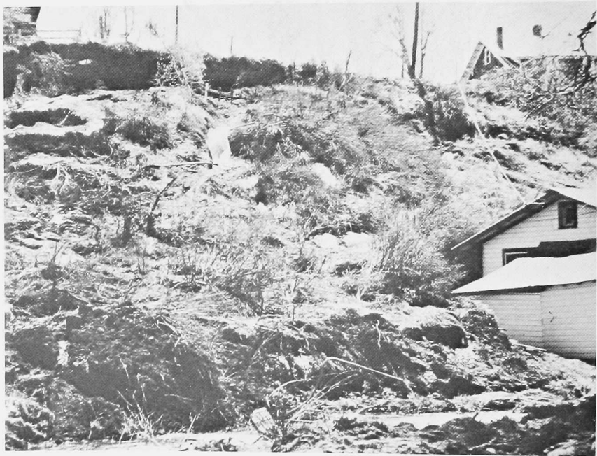
Figure 10. A LANDSLIDE IN A RESIDENTIAL AREA THAT HAS DAMAGED SEVERAL BUILDINGS. NOTE THE CROWN, MAIN SCARP, AND OTHER FEATURES OF THE LANDSLIDE (SEE FIGURE 6).
