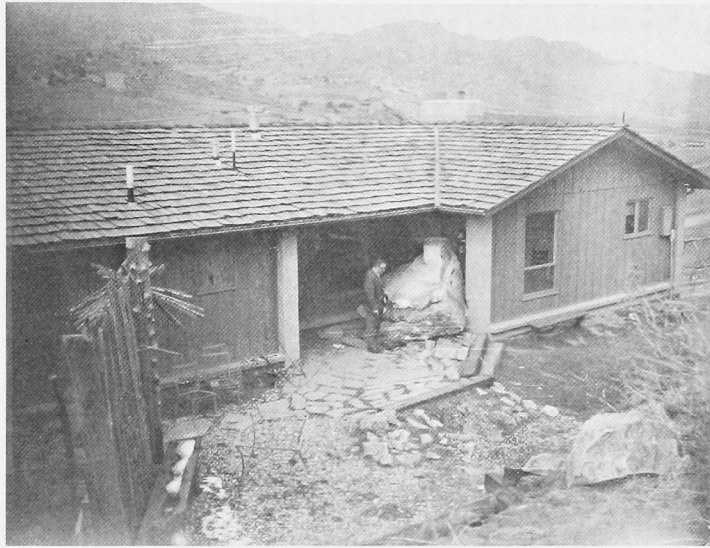
Figure 15. A BLOCK OF ROCK ROLLED DOWNHILL AND DAMAGED THIS HOUSE. WHAT MIGHT HAVE HAPPENED IF THE ROCK HAD BEEN LARGER OR IF IT HAD ROLLED DOWN A STEEPER SLOPE?
