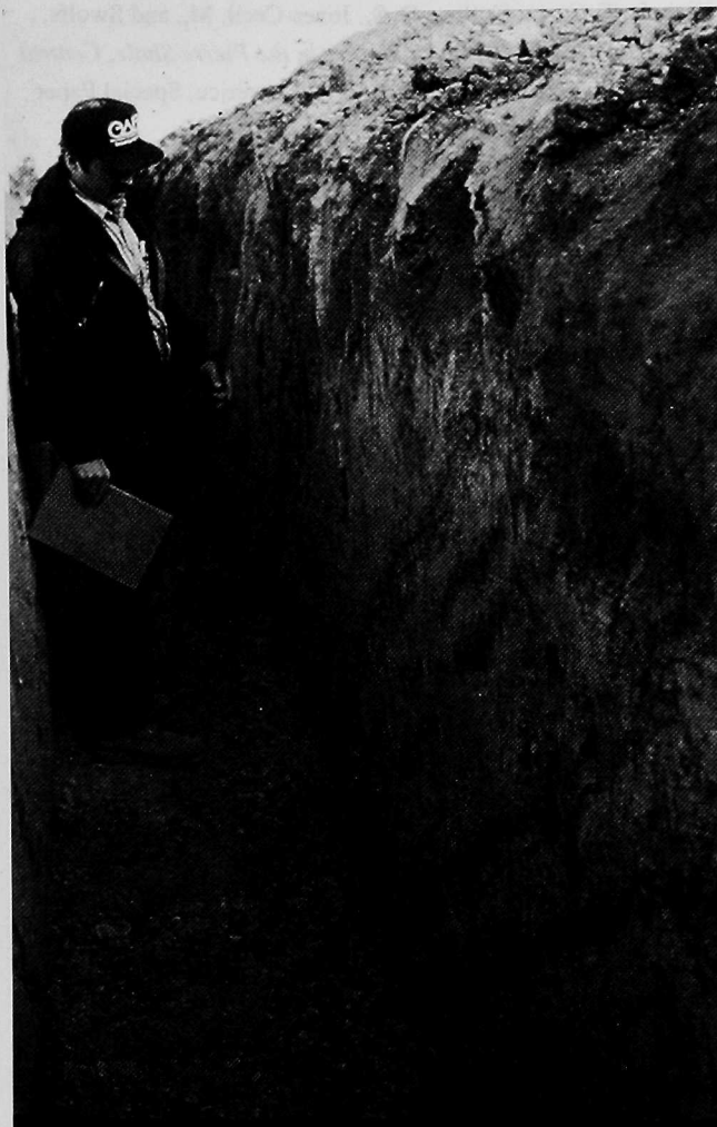
FIGURE 9: This trench has exposed dipping beds of bentonite (dark layers) at a high school site. Earlier drillhole surveys had not encountered the bentonite. The foundation design for the school was subsequently changed from a drilled-pier system to an overexcavation design.
