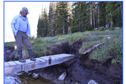
Ditch diverts groundwater flow from fen to reservoir
