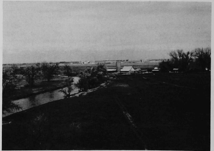
Figure 9. Existing land-use conflicts between farm land, gravel deposits, and industrialization in the flood plain of the Cache la Poudre River. View to the northwest across the Cache la Poudre River flood plain toward the Kodak plant, Weld County. Photograph by W. P. Rogers, Colorado Geological Survey.
