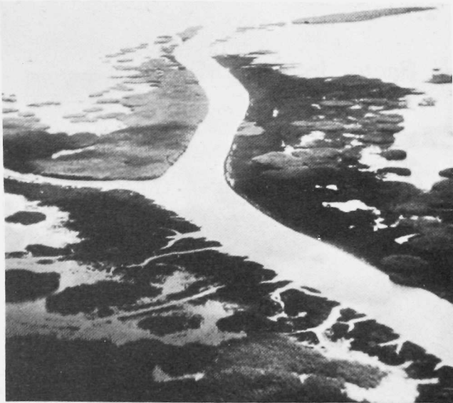
Figure 1.--Distributary channels in the lower delta plain of the Mississippi Delta. Observe the numerous breaches in the poorly developed levees of the distributary channels. (Photo courtesy of R. S. Saxena.)
