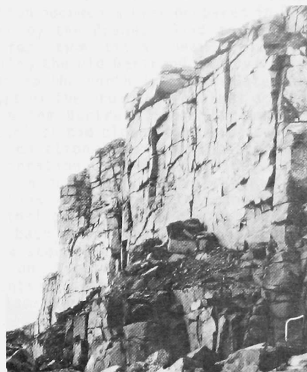
Figure 6. Top, southwestward view of the Rogers quarry on the west rim of North Table Mountain. Bottom, on the old quarry wall, notice how columnar jointing in the latite flow stabilizes the cut on the vertical face. Western Paving Construction Company plans to expand the old quarry eastward.
