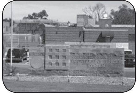
La Vista Correctional Facility
