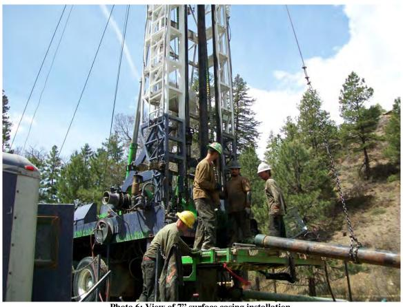
Photo 6: View of 7" surface casing installation.
