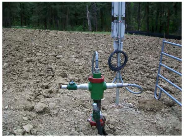
Photo 12: View of well head and telemetry equipment at the Deep Canyon site.
