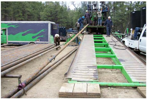
Photo 8: View of 4.5" long string casing installation..
