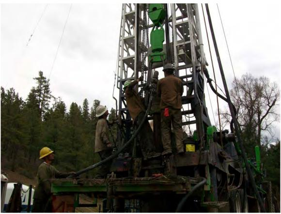
Photo 7: View of the cementing operations for the 7" surface casing.
