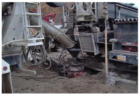
Photo 7: View of cementing of the 4.5" casing at the BP Highlands site.
