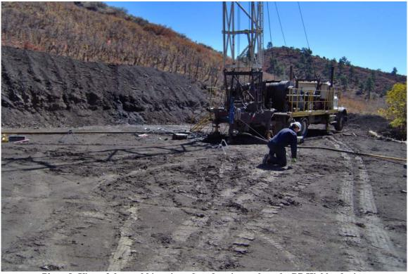
Photo 8: View of the swabbing rig and perforating tools at the BP Highlands site.
