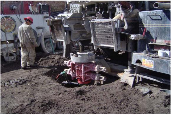
Photo 12: View of View of Blow-Out Preventer at the Fiddler site.
