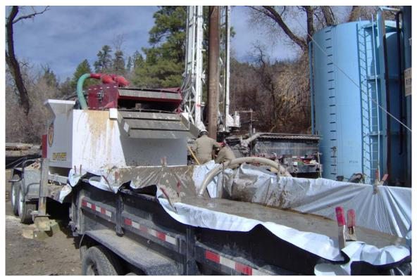
Photo 15: View of conductor casing installation at the Palmer
