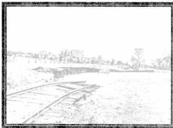
1957 Flood - Railroad washout near Lyons.
