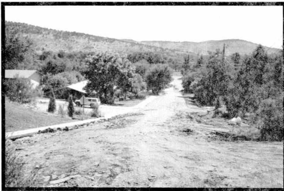
Flood waters caused erosion to Prospect St., west of town.
