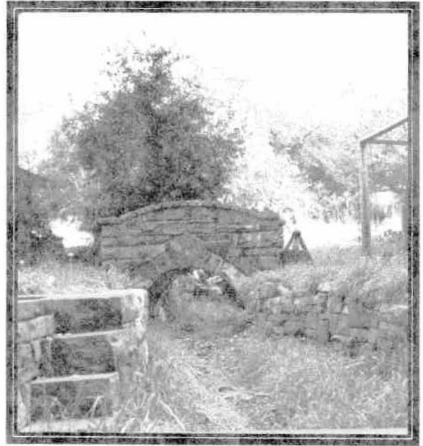
Lyons drainage ditch: photo taken at property on Reese Street.
