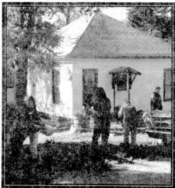
NCCC workers cleaning ditch in front of flooded property.
